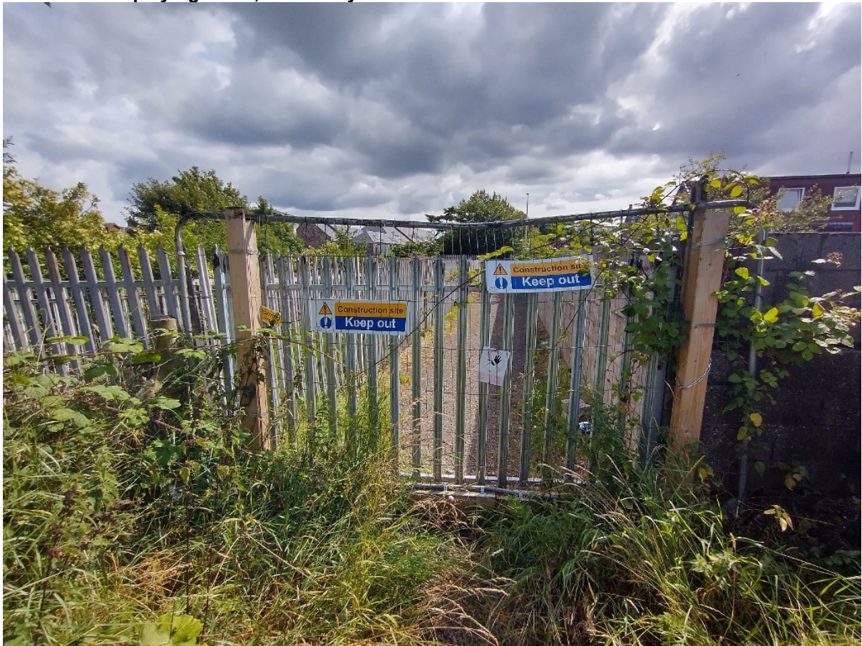
The fencing is unaltered from 2020. The path in the foreground has become partially overgrown with vegetation.
