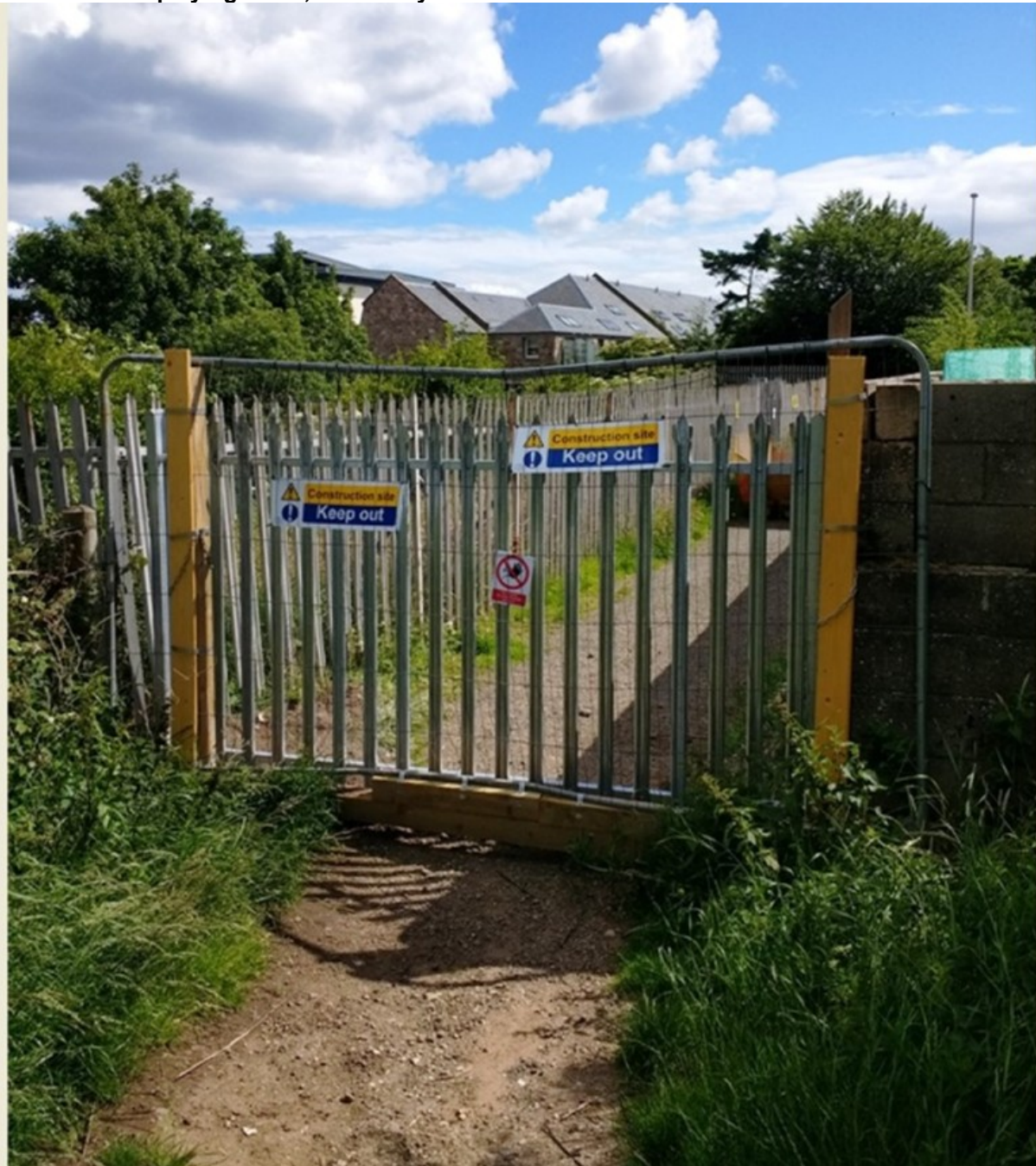
The entrance from the playing fields has been closed with a 'Heras' type temporary security panel supported by sturdy wooden posts. There are signs on the fence panel stating, 'construction site, keep out'. Behind the fence panel there is a metal palisade fence approximately 1.8 metres high, of similar construction to the fence that surrounds the adjacent electricity sub-station. In the foreground, within the public park, there is well-worn earth path approximately 1 metre wide.
