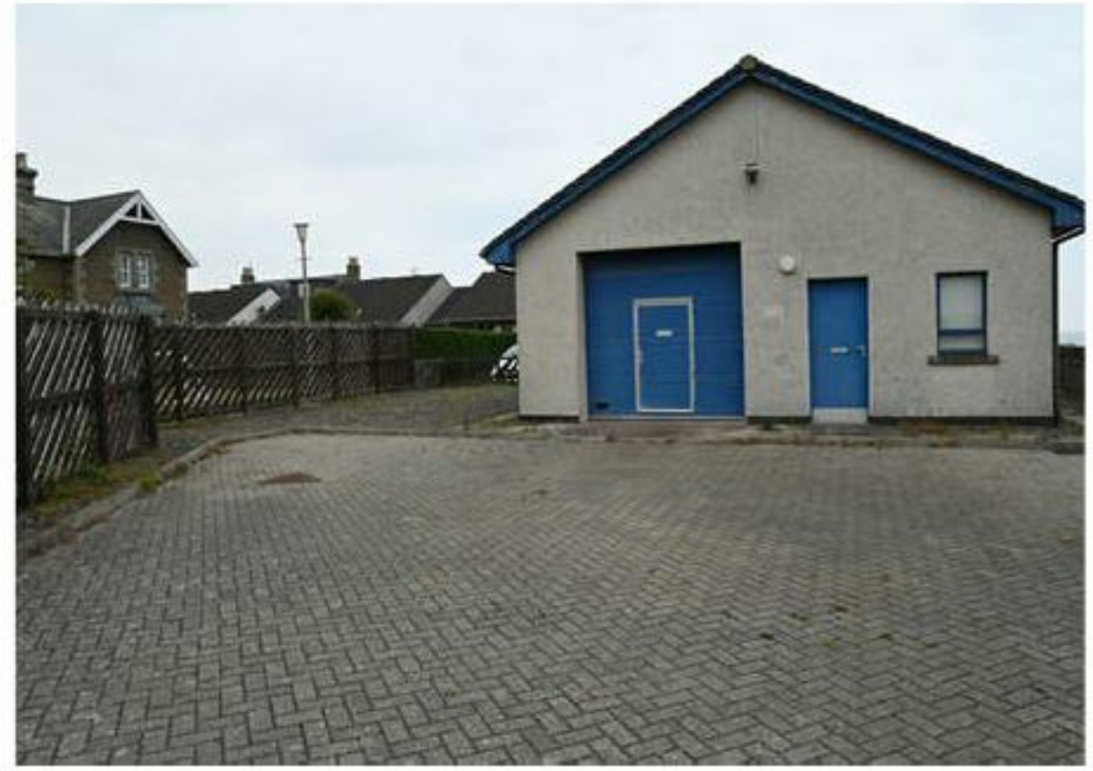
Coastguard Station & existing boundary
