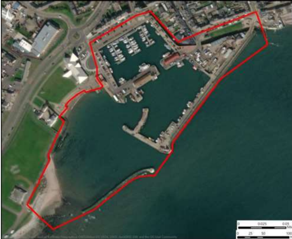
Figure 3 Limits Shown on Aerial image
