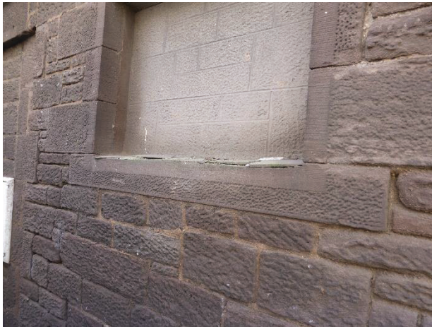
101 Delaminating sill
