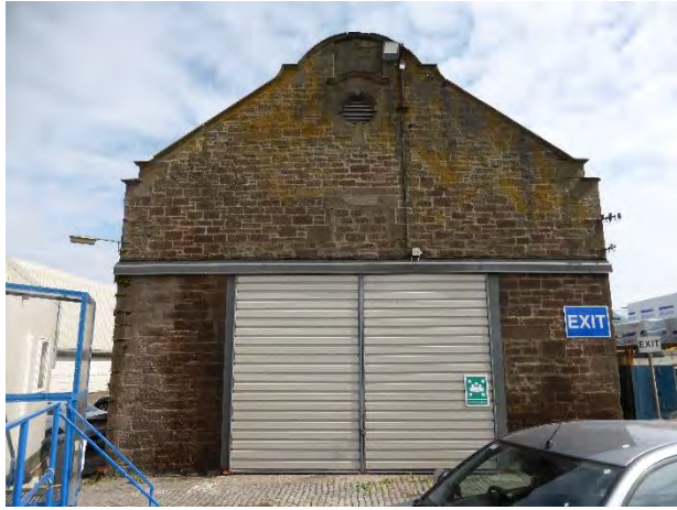
SW elevation (gable)
