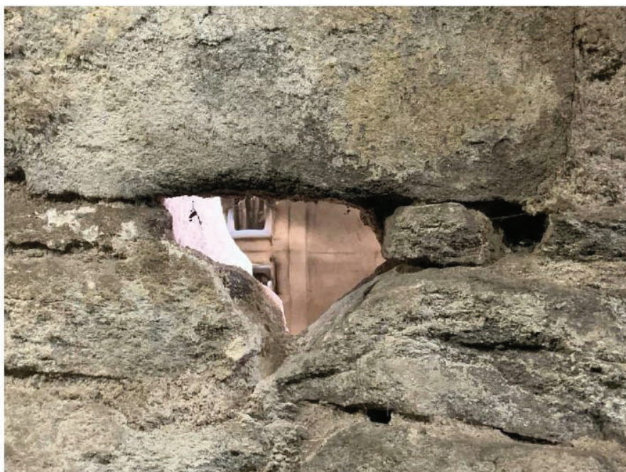
Figure 28: Damaged Stonework
