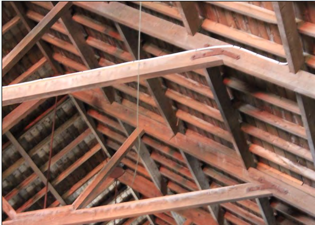
Figure 8. Slates laid onto wooden sarking and joists.
