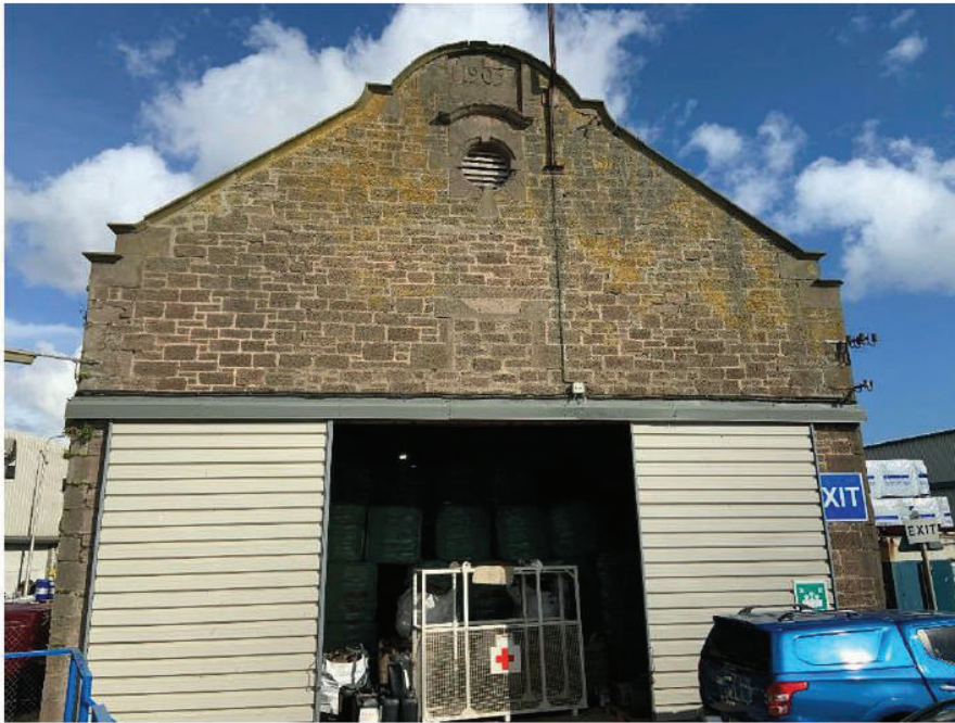
Figure 1: South West Gable Elevation
