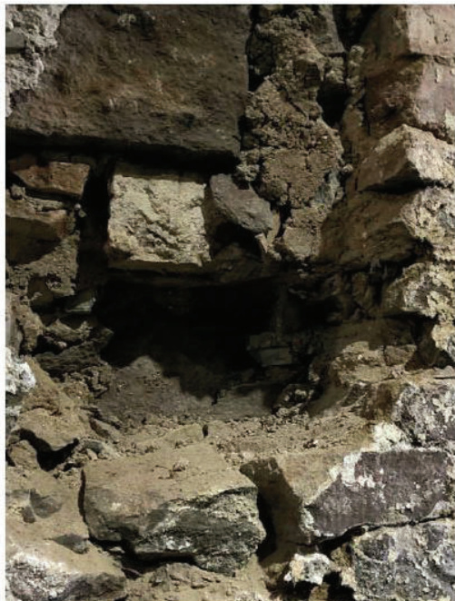
Figure 27: Damaged Stonework
