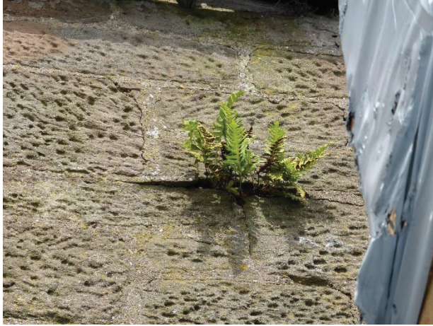
163 Vegetation + spalling
