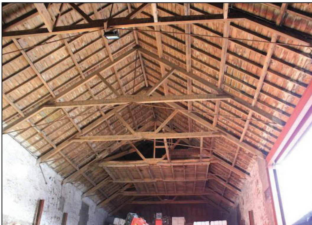
Figure 5. Warehouse actively used for storage with open doors during working hours.
