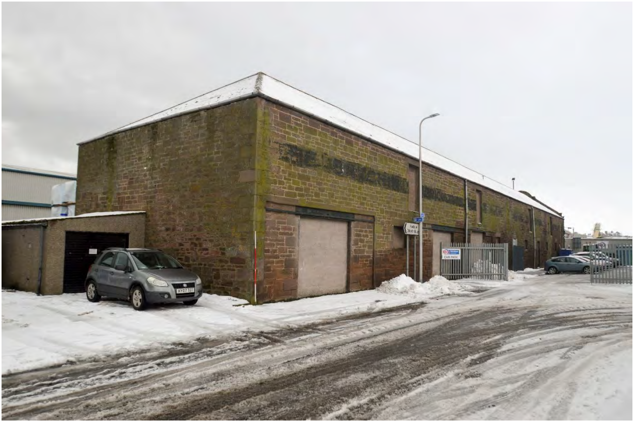
Illus 6 General view looking S along the NE/NW exterior.
