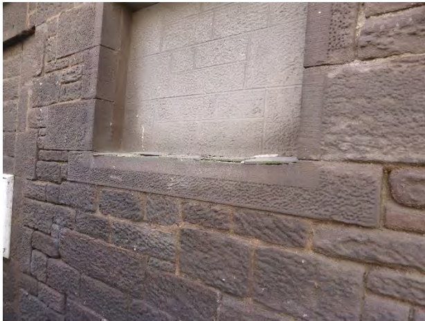
101 Delaminating sill
