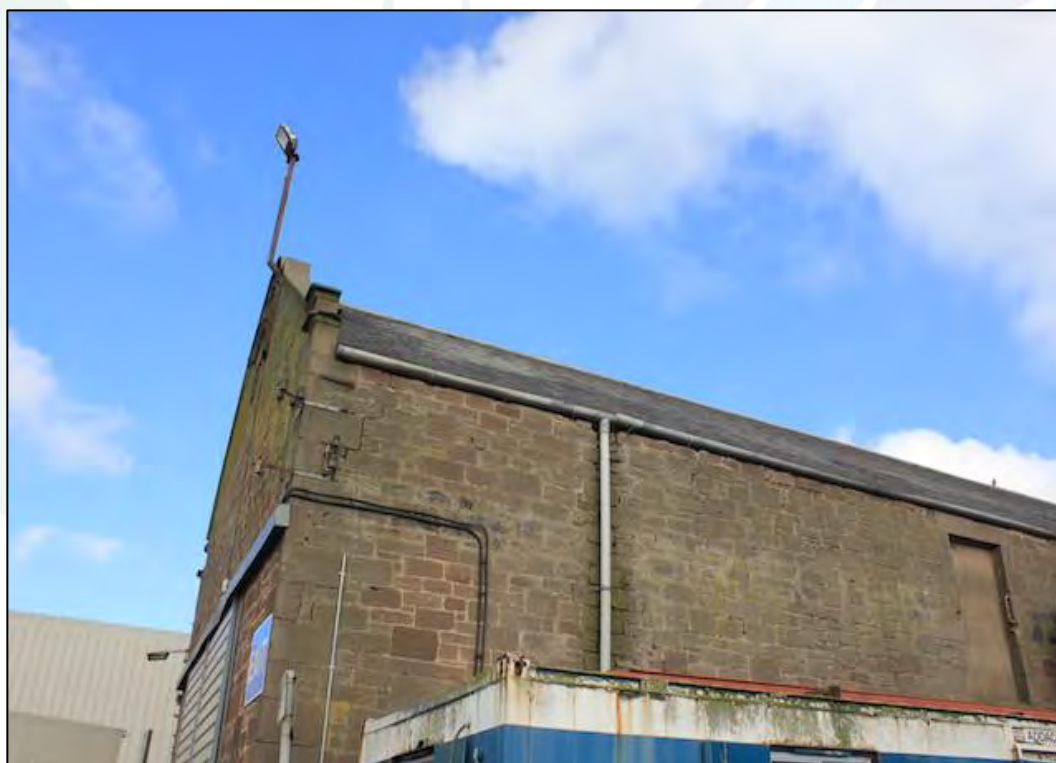
Figure 2. Stonework construction of warehouse.
