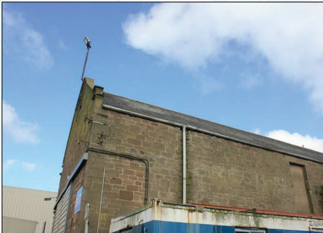
Figure 2. Stonework construction of warehouse.
