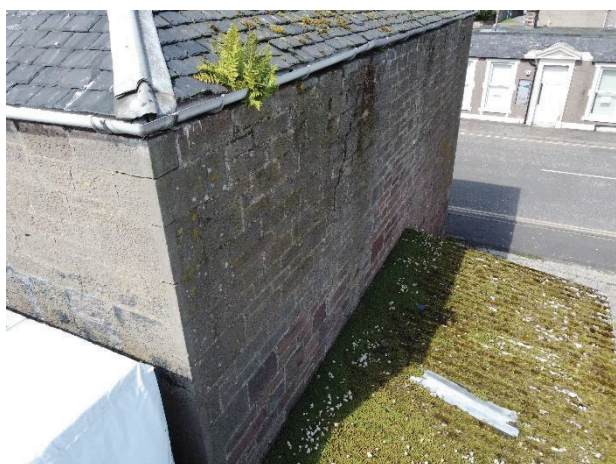
Outwards leaning of the wall
