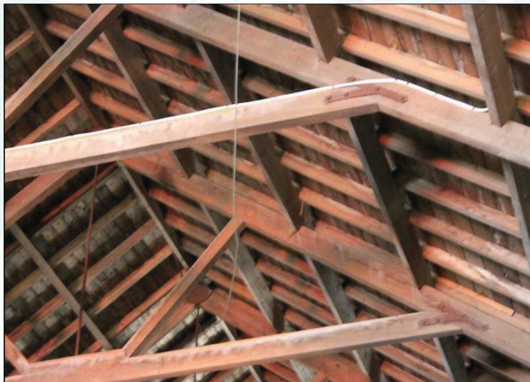
Figure 8. Slates laid onto wooden sarking and joists.
