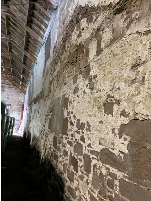
Figure 17: Internal South West Elevation –Wall Lean, Weathered Stone, Patches & Cracking
