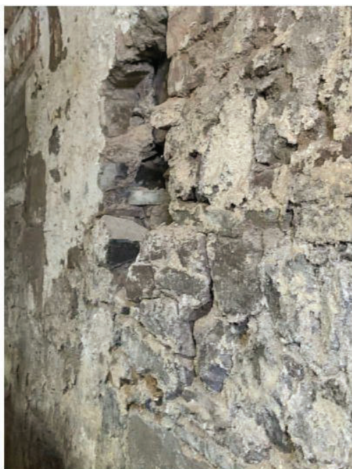
Figure 26: Damaged Stonework
