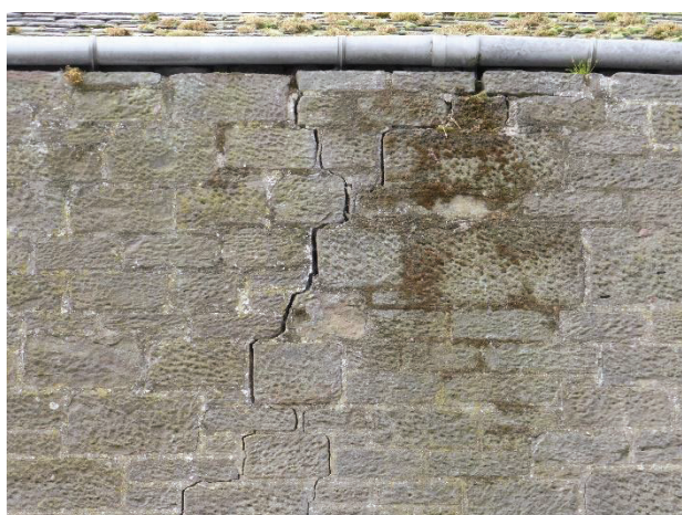
Structural movement cracks
