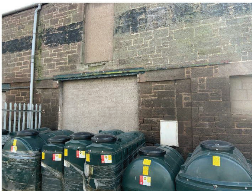
Figure 8: North West Elevation – Altered Openings, Damp Pathces & Eroded Stone and Mortar
