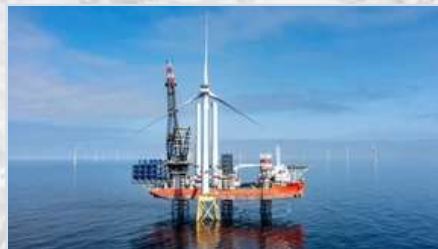
Final wind turbine installed
