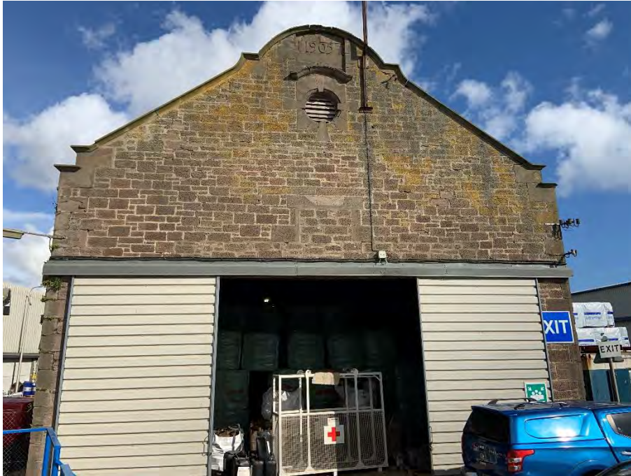
Figure 1: South West Gable Elevation
