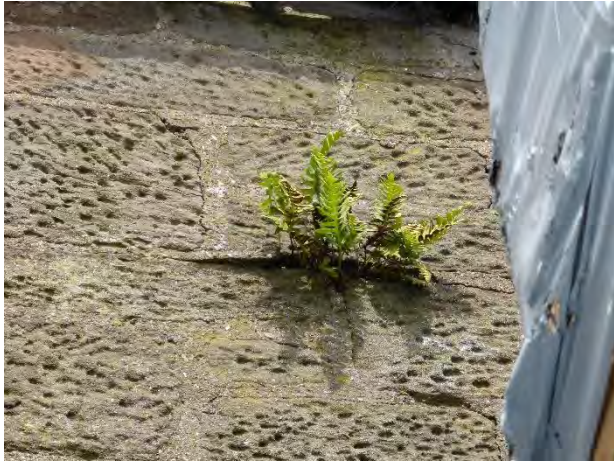
163 Vegetation + spalling
