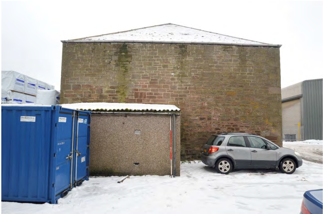
Illus 13 NE facing exterior with small modern garage addition.
