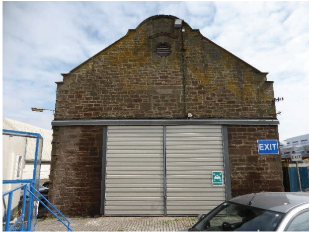
SW elevation (gable)
