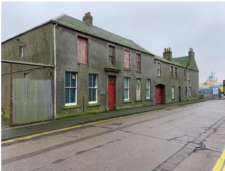
Photograph 2.01 America Street Offices - External Elevation
