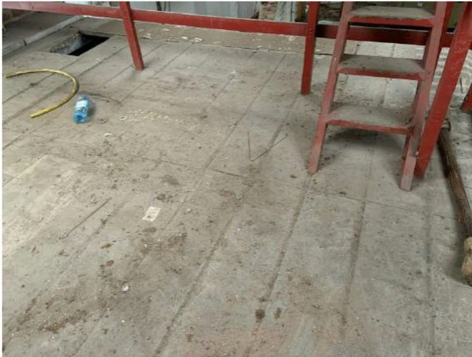
Photograph 4.07 - New Workshop/Store – Precast Ceiling/Floor
