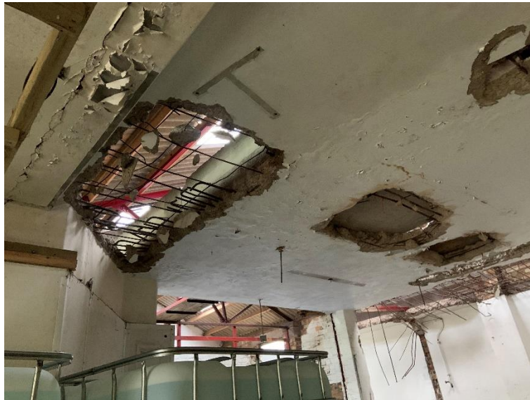
Photograph 4.09 - New Workshop/Store – Reinforced Concrete/Floor
