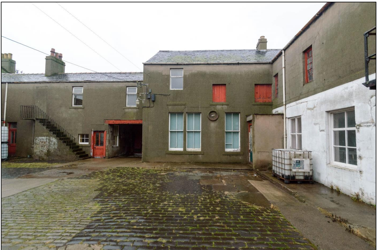
Illus 13 General view of NW and NE courtyard elevations.
