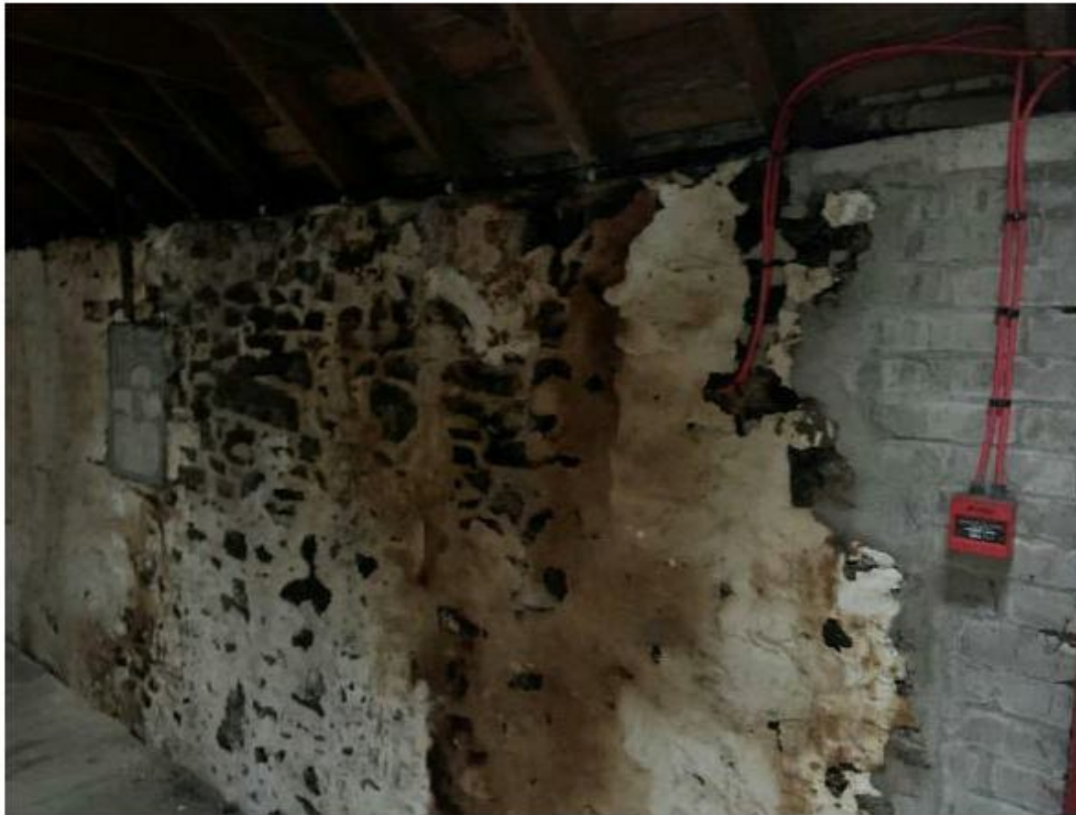
Photograph 3.20 - Old Workshop/Store –California Street Wall
