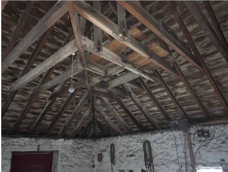
Photograph 2.02 America Street Offices – Roof Internal
