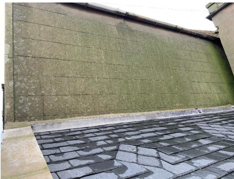
Photograph 3.03 - Old Workshop/Store – California Street Elevation
