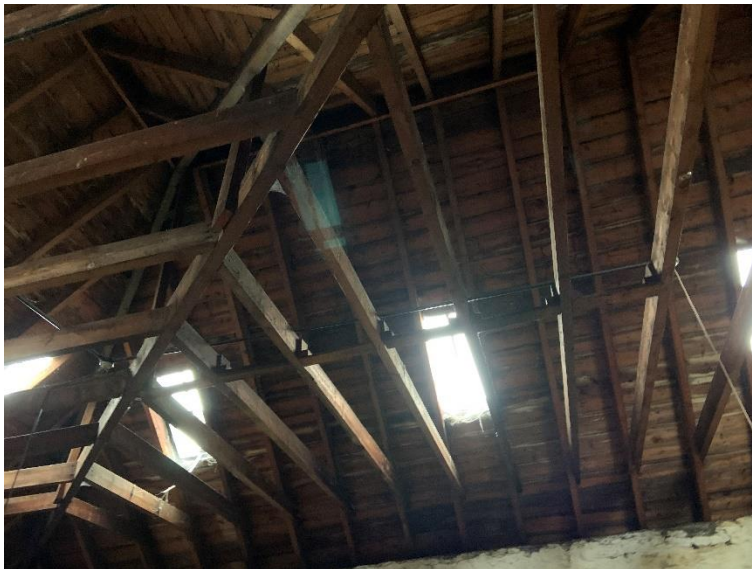
Photograph 3.19 - Old Workshop/Store –California Street Roof
