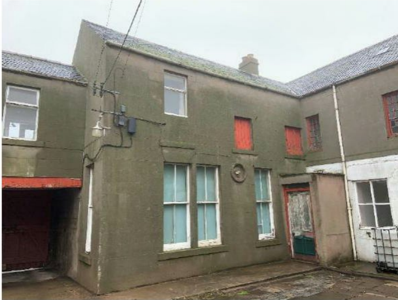
Photograph 2.10 America Street Offices - Quadrangle External Elevation – Section 2b
