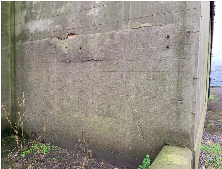
Photograph 4.04 - New Workshop/Store – Return to Managers Office
