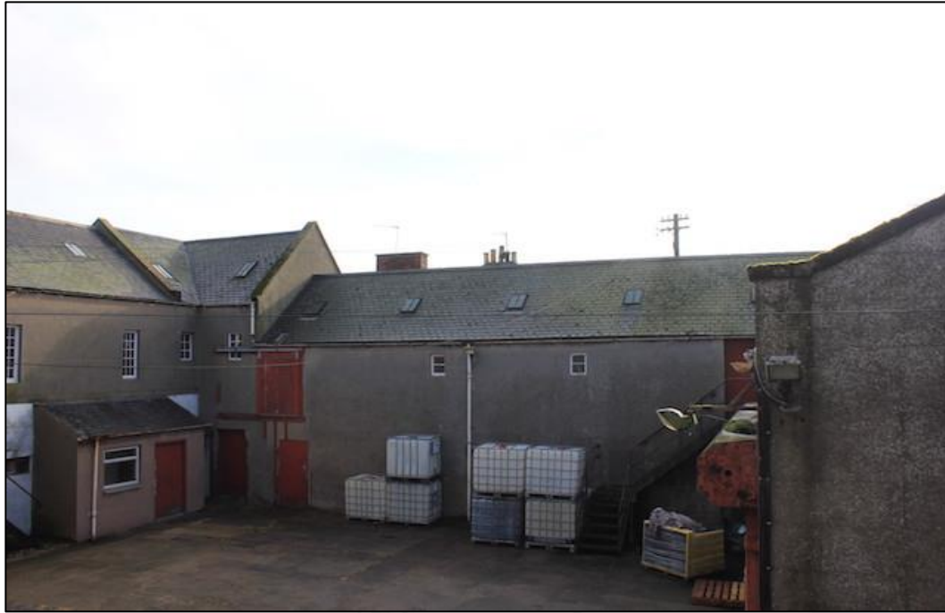
Figure 8. Interior courtyard to be demolished.
