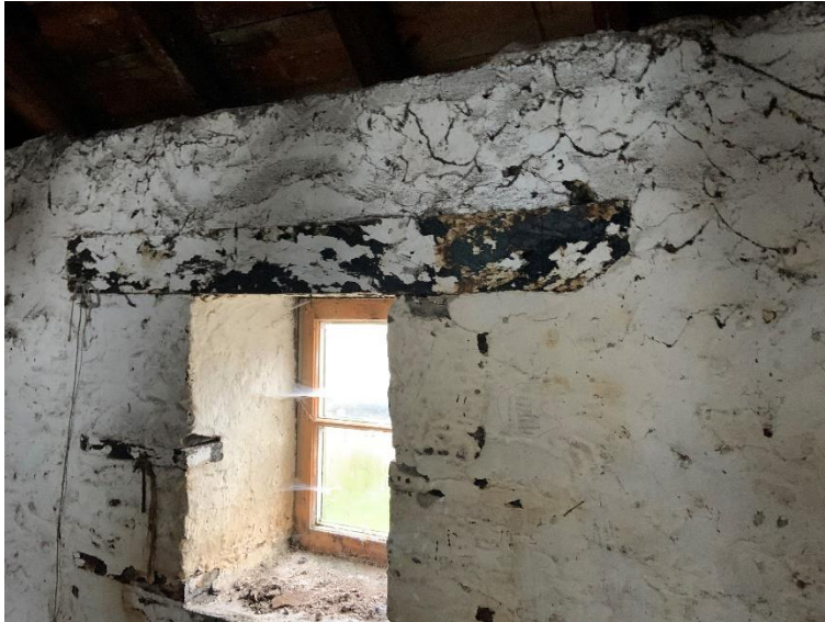
Photograph 3.22 - Old Workshop/Store –California Street Wall Lintel
