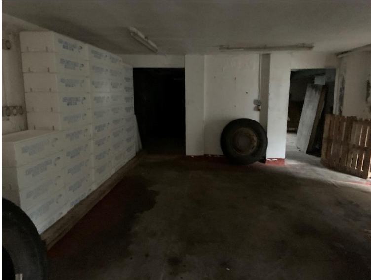
Photograph 3.08 - Old Workshop/Store – Ground Floor
