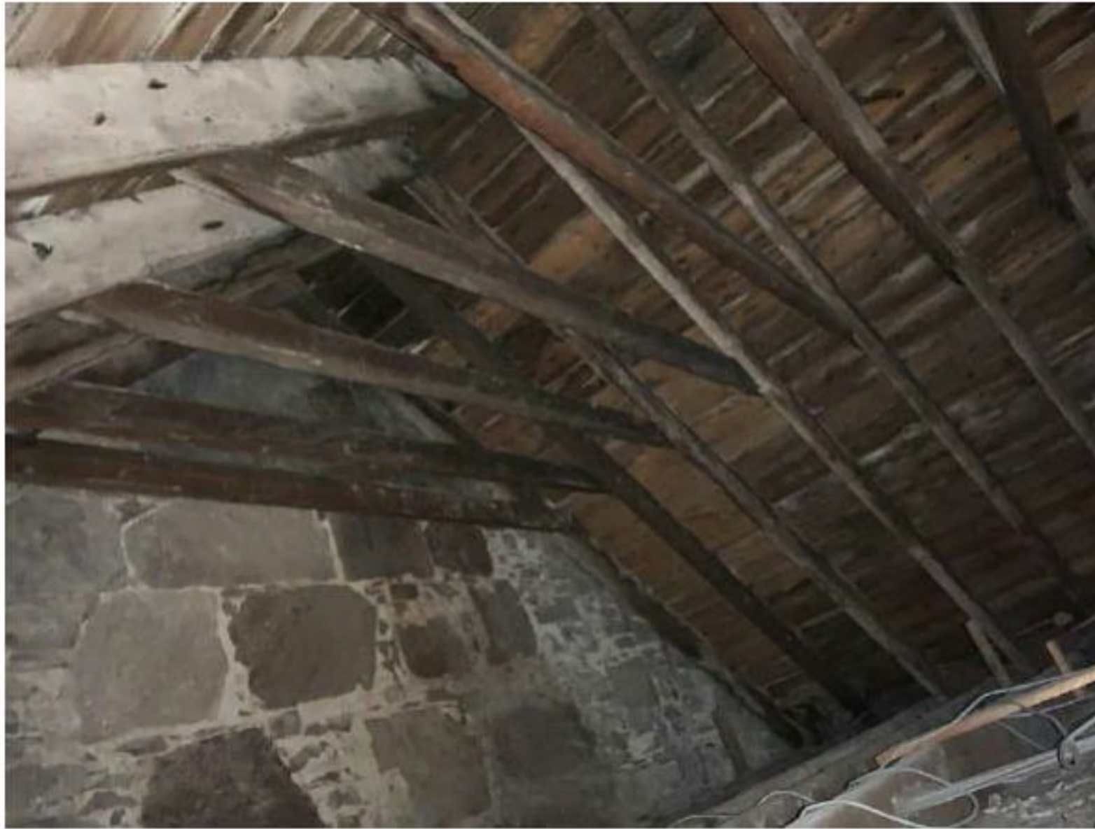
Photograph 1.02 Managers House – Roof Trusses
