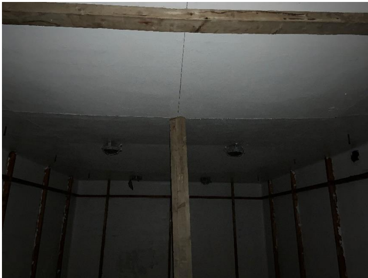
Photograph 3.13 - Old Workshop/Store – Specialist Room 2
