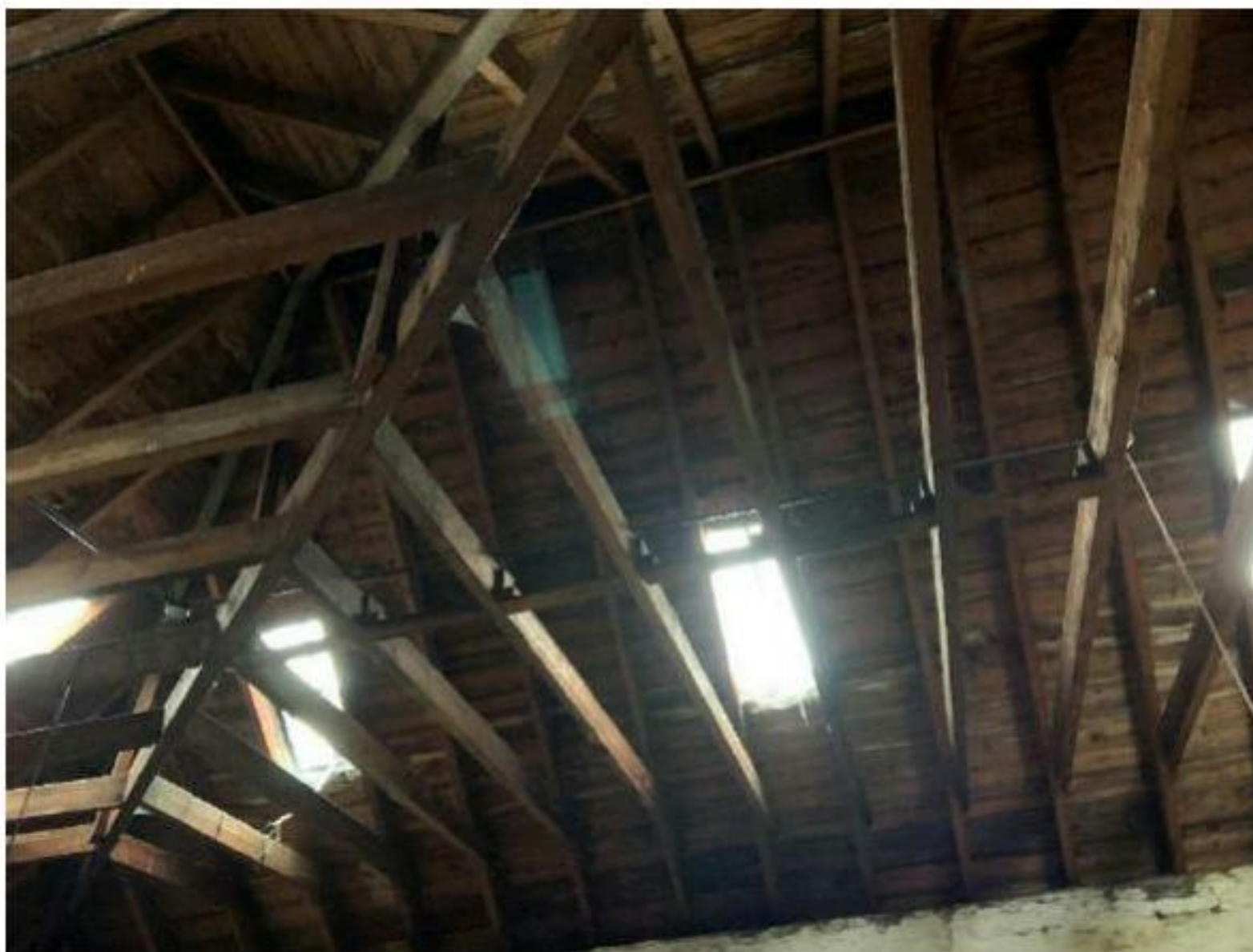
Photograph 3.19 - Old Workshop/Store –California Street Roof
