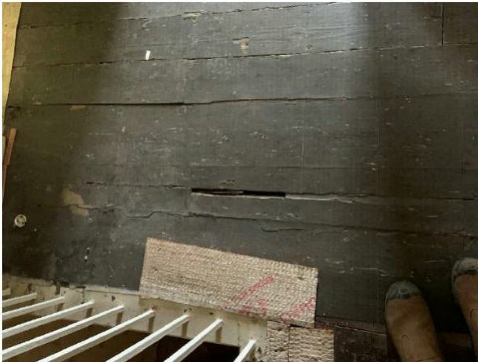
Photograph 1.07 Managers House – 1 st Floor
