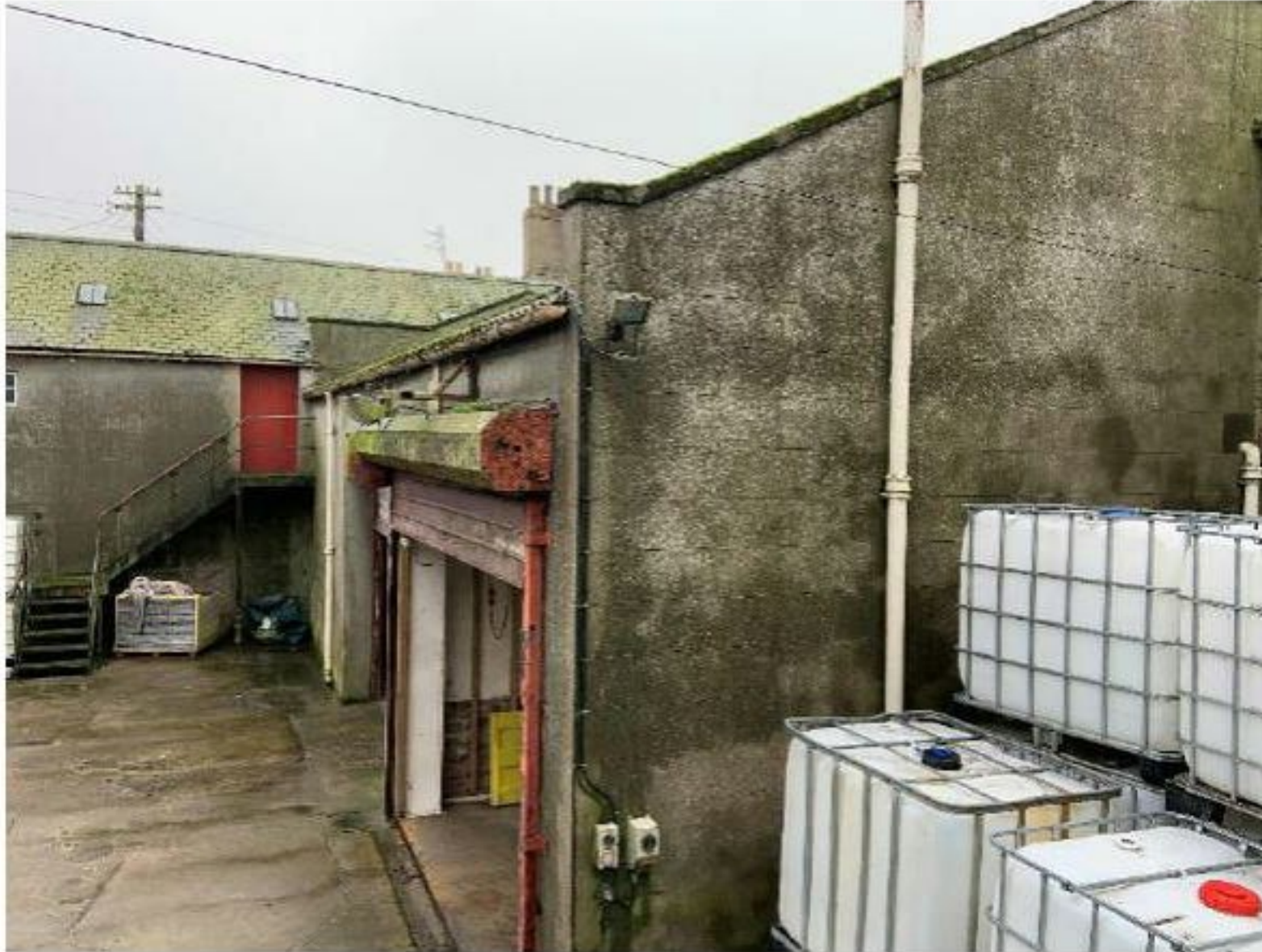
Photograph 4.05 - New Workshop/Store – Quadrangle Opening
