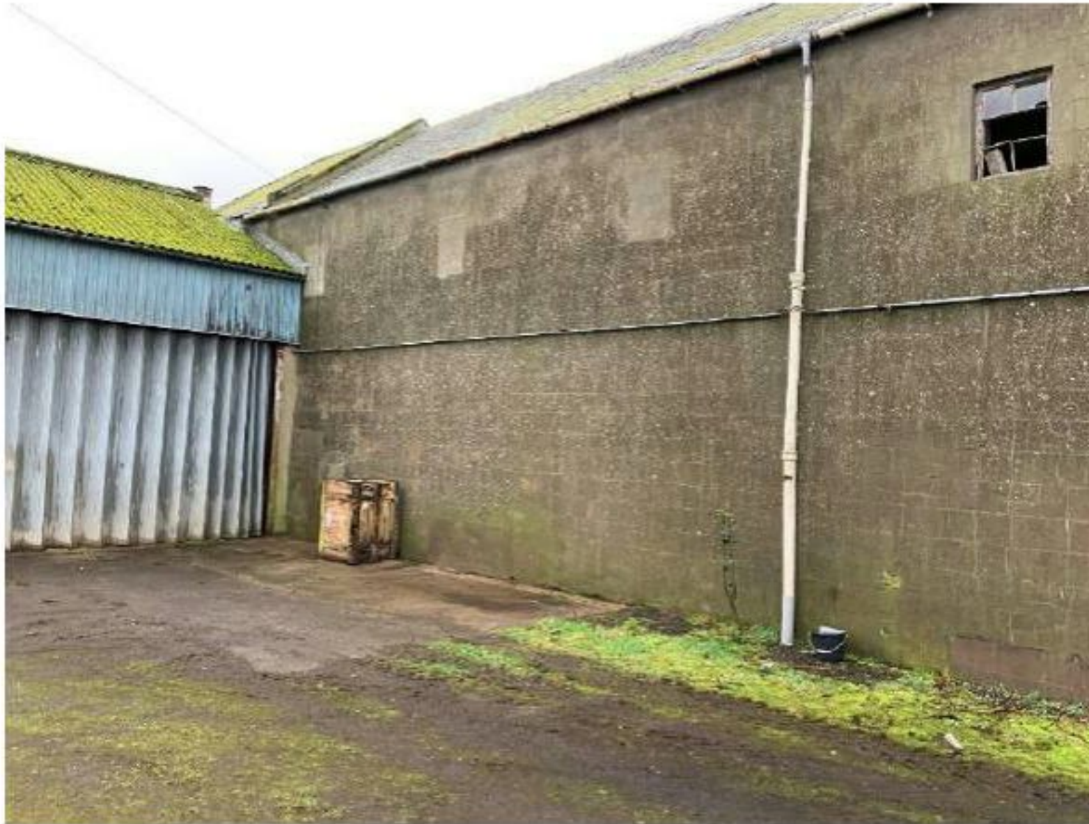
Photograph 3.01 Old Workshop/Store – Rear Elevation
