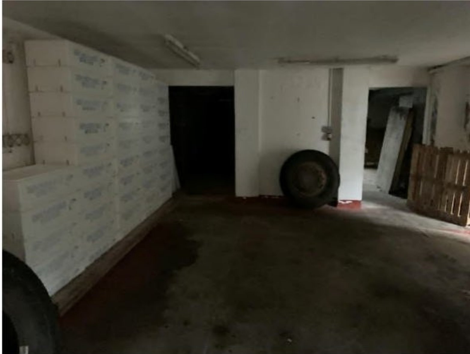
Photograph 3.08 - Old Workshop/Store – Ground Floor
