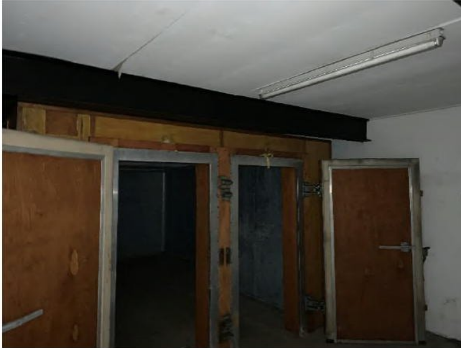
Photograph 3.12 - Old Workshop/Store – Specialist Room 1
