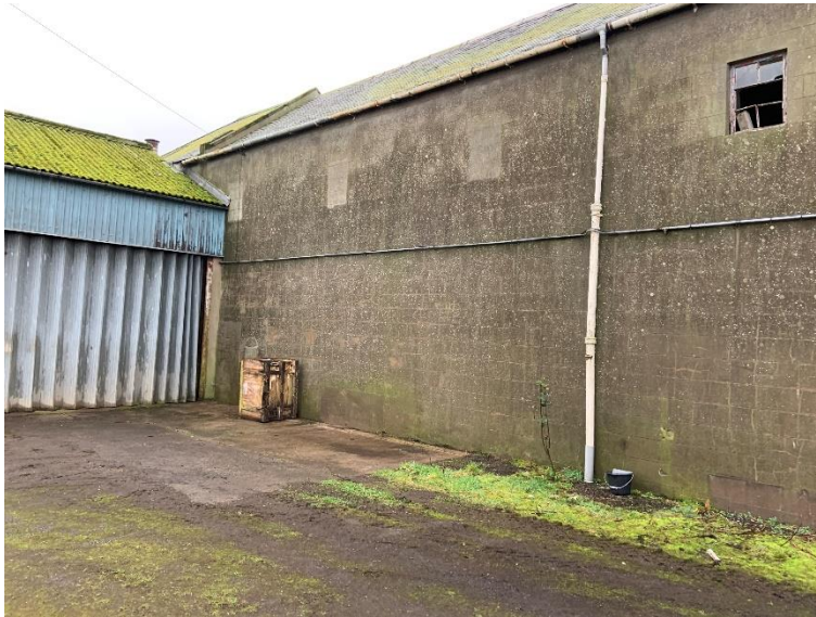
Photograph 3.01 Old Workshop/Store – Rear Elevation
