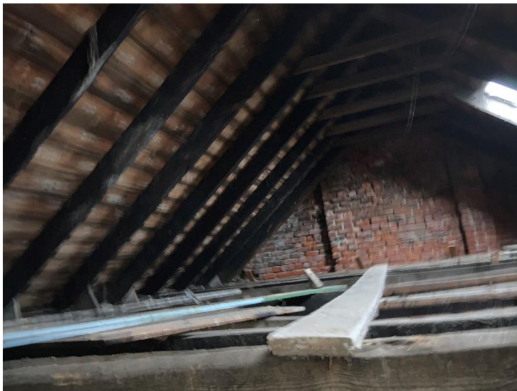
Photograph 3.02 - Old Workshop/Store - Roof
