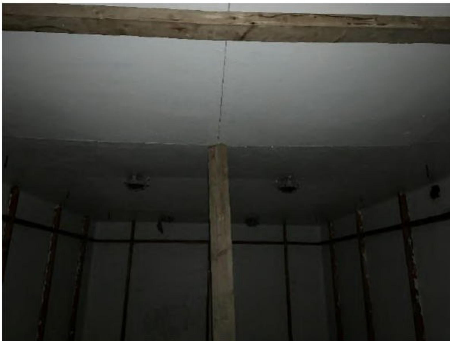
Photograph 3.13 - Old Workshop/Store – Specialist Room 2
