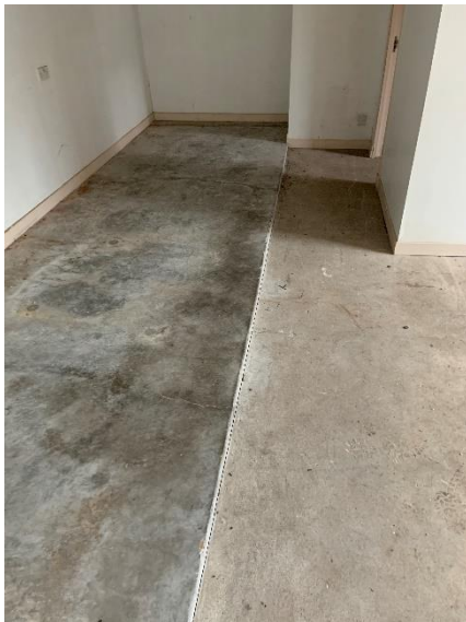
Photograph 3.07 - Old Workshop/Store – Ground Floor
