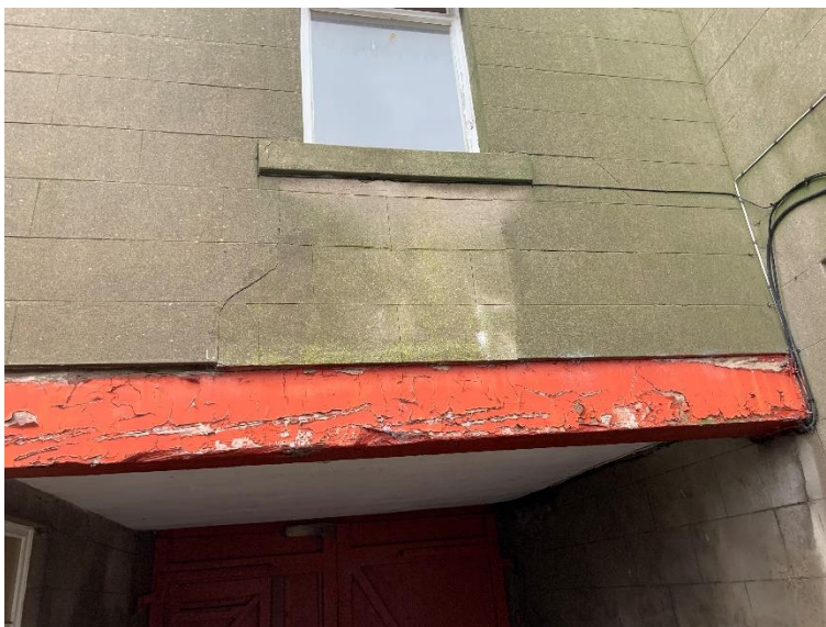
Photograph 2.07 America Street Offices - Quadrangle External Elevation – Arch Lintel
