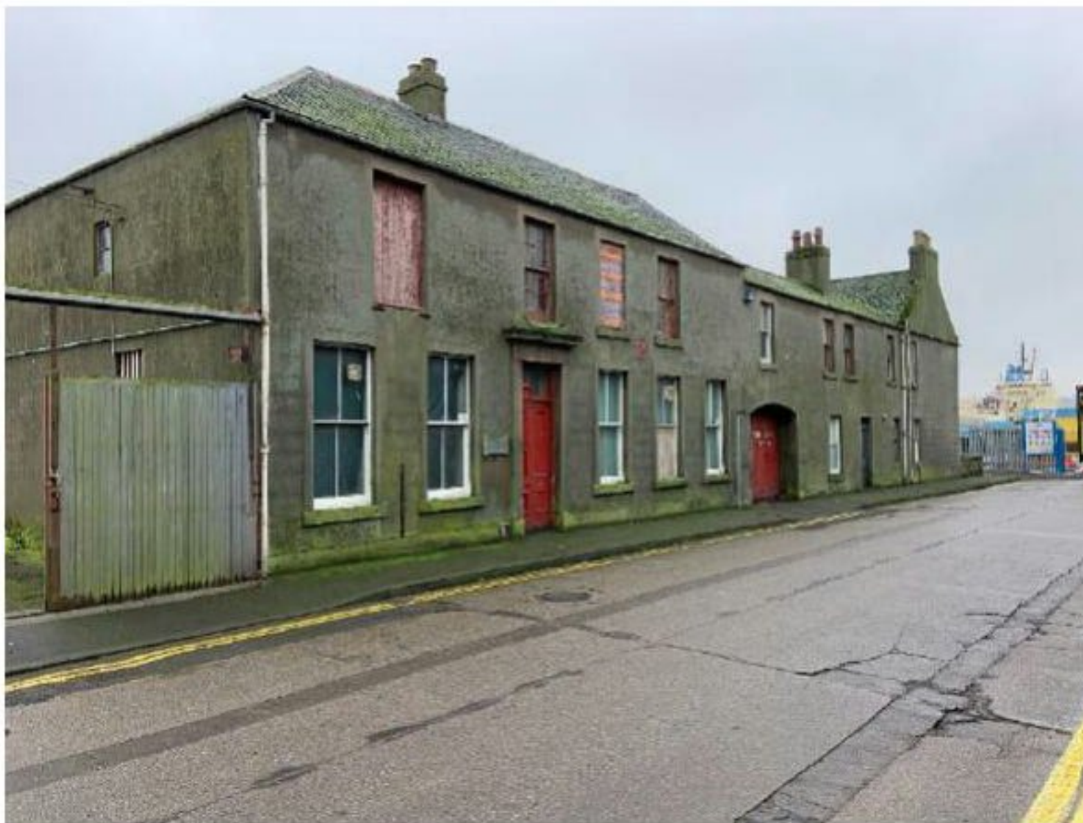
Photograph 2.01 America Street Offices - External Elevation
