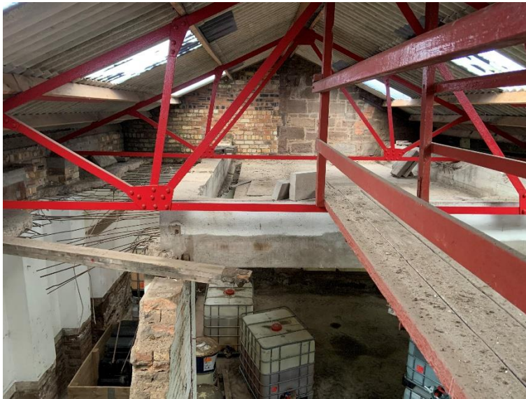
Photograph 4.02 - New Workshop/Store - Roof
