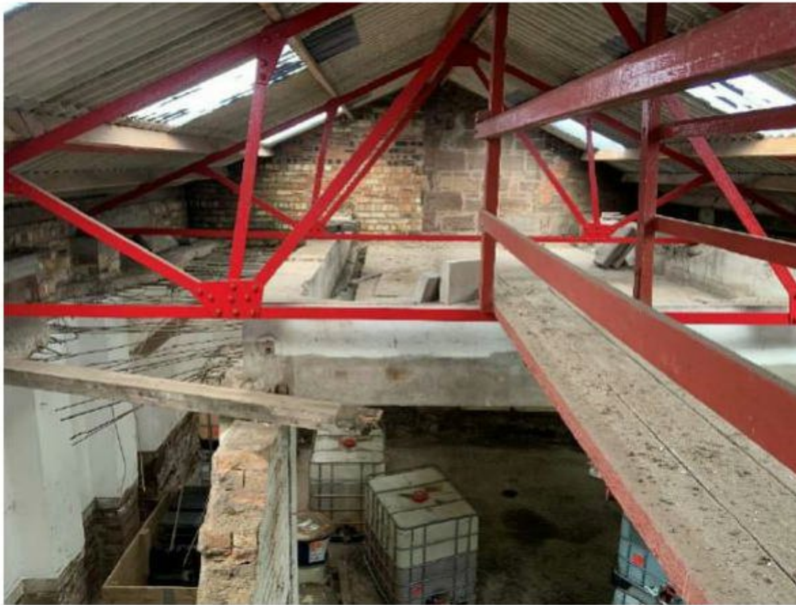
Photograph 4.02 - New Workshop/Store - Roof
