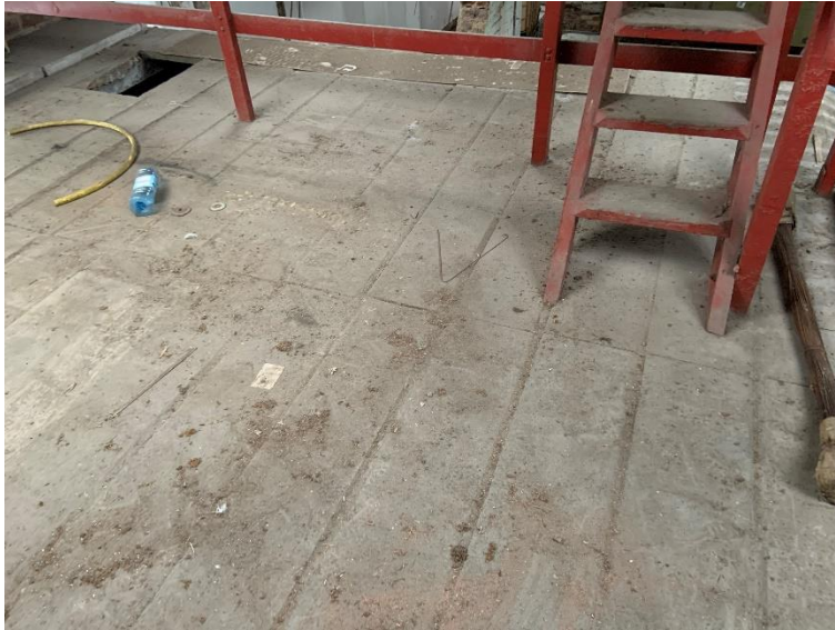
Photograph 4.07 - New Workshop/Store – Precast Ceiling/Floor
