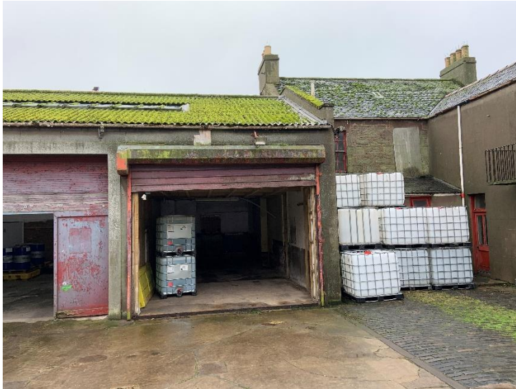
Photograph 1.06 Managers House - External Wall – Rear Elevation
