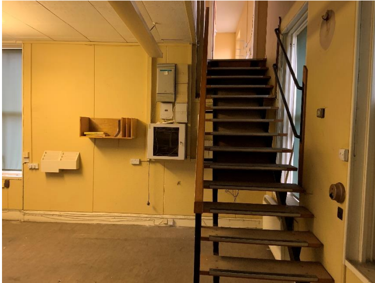
Photograph 2.12 America Street Offices – Internal - Stairs
