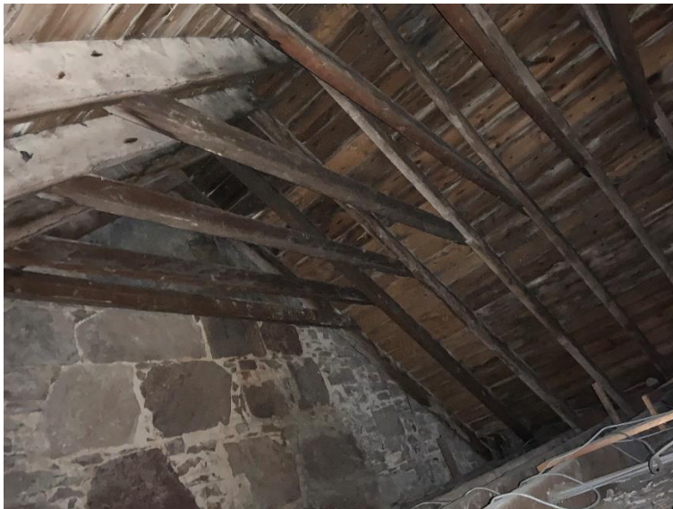
Photograph 1.02 Managers House – Roof Trusses
