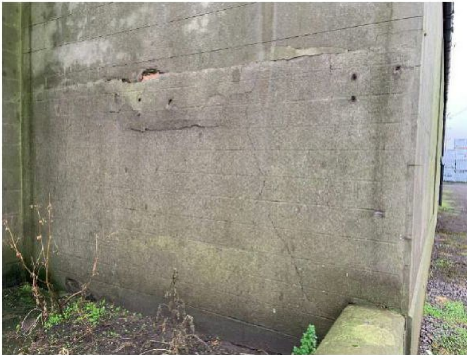
Photograph 4.04 - New Workshop/Store – Return to Managers Office
