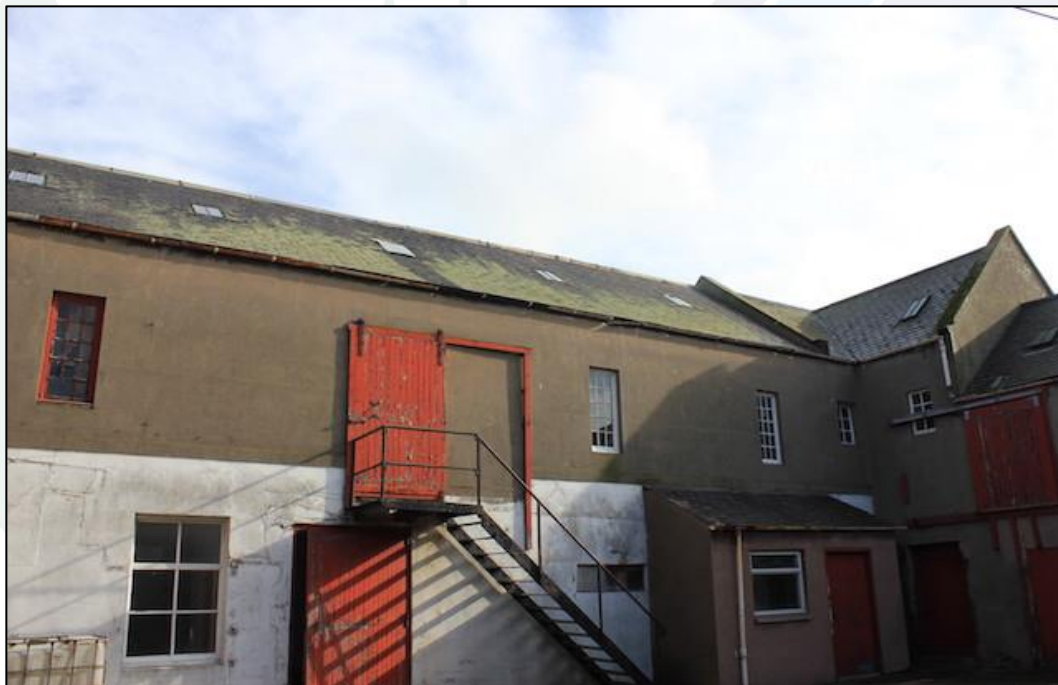
Figure 9. Interior courtyard to be demolished.
