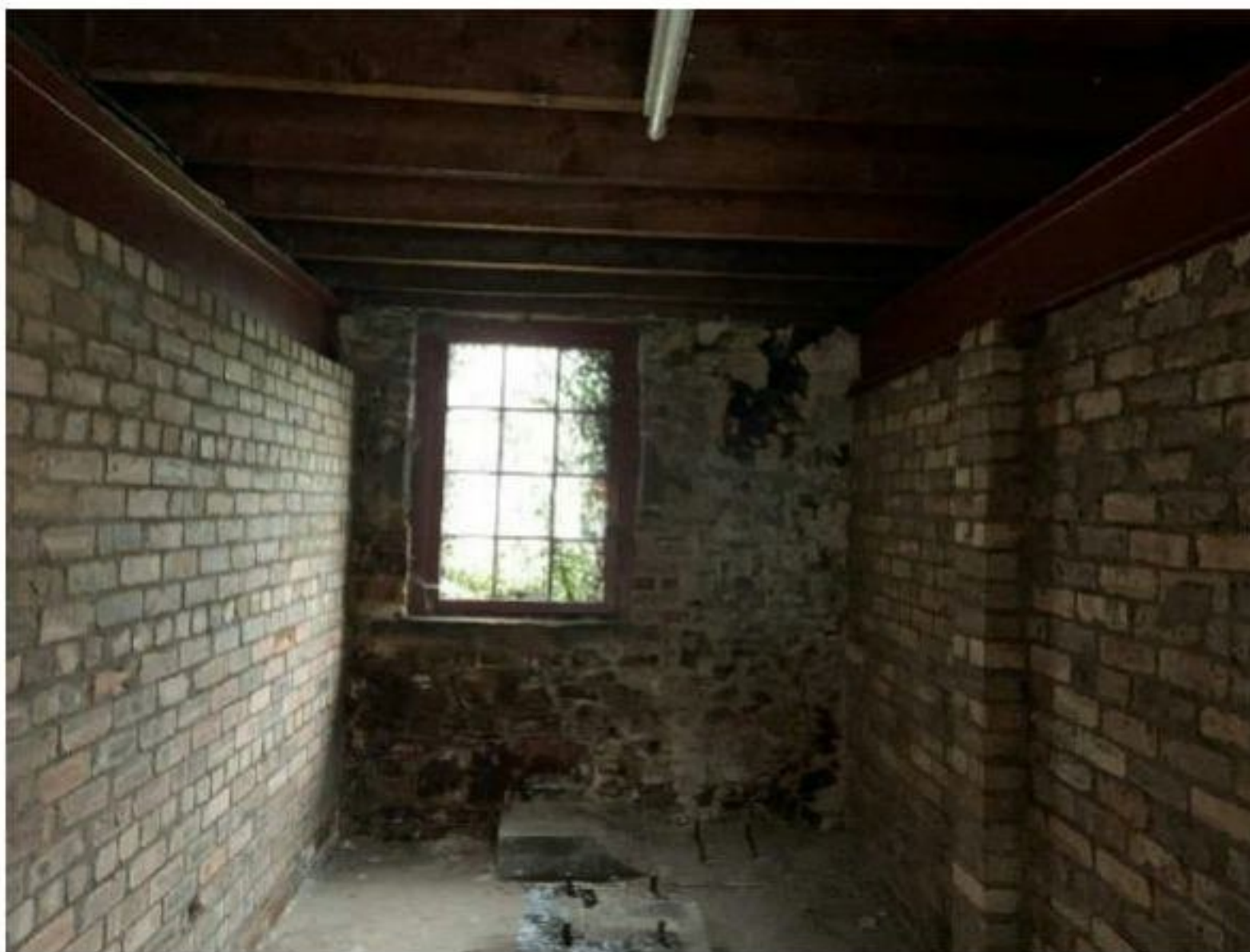
Photograph 3.11 - Old Workshop/Store – Steel Beams / Brick Walls / Floor Joists
