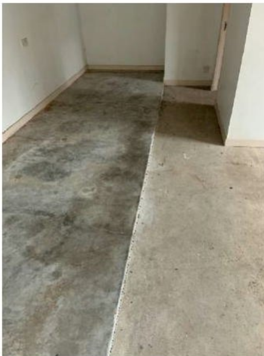
Photograph 3.07 - Old Workshop/Store – Ground Floor
