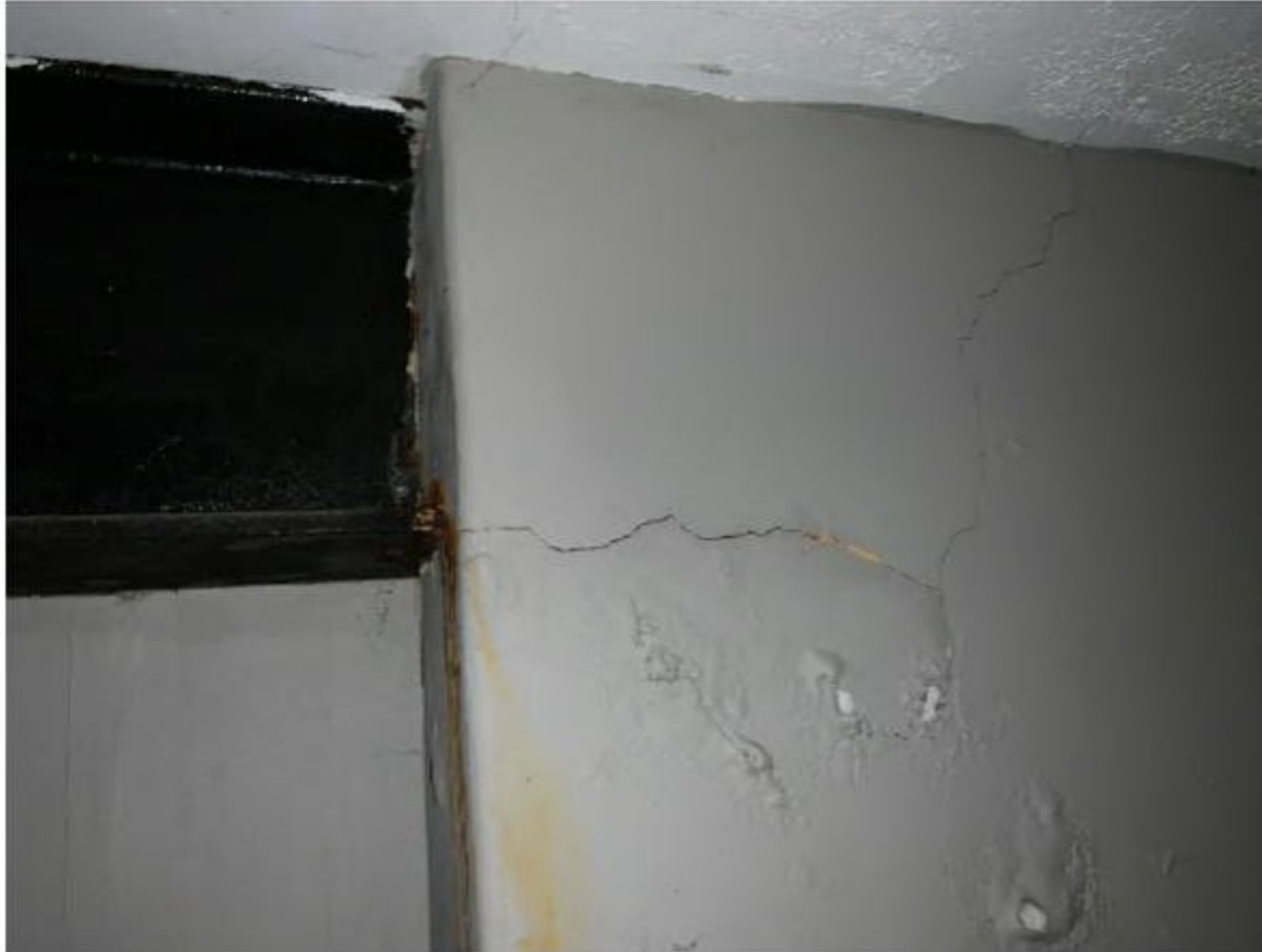
Photograph 3.10 - Old Workshop/Store – Steel Beams Support
