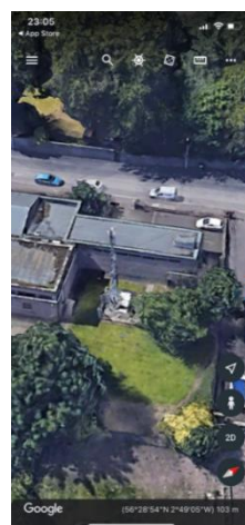
BT Mast at the bottom of Victoria Street
