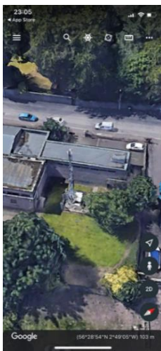
BT Mast at the bottom of Victoria Street with ample ground space.
