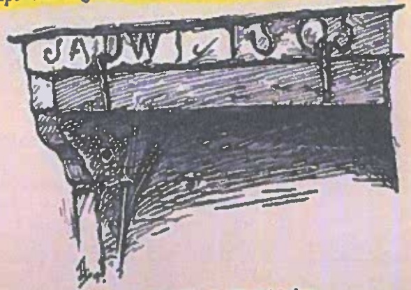
Fireplace Lintel, Old Gairie Inn.
