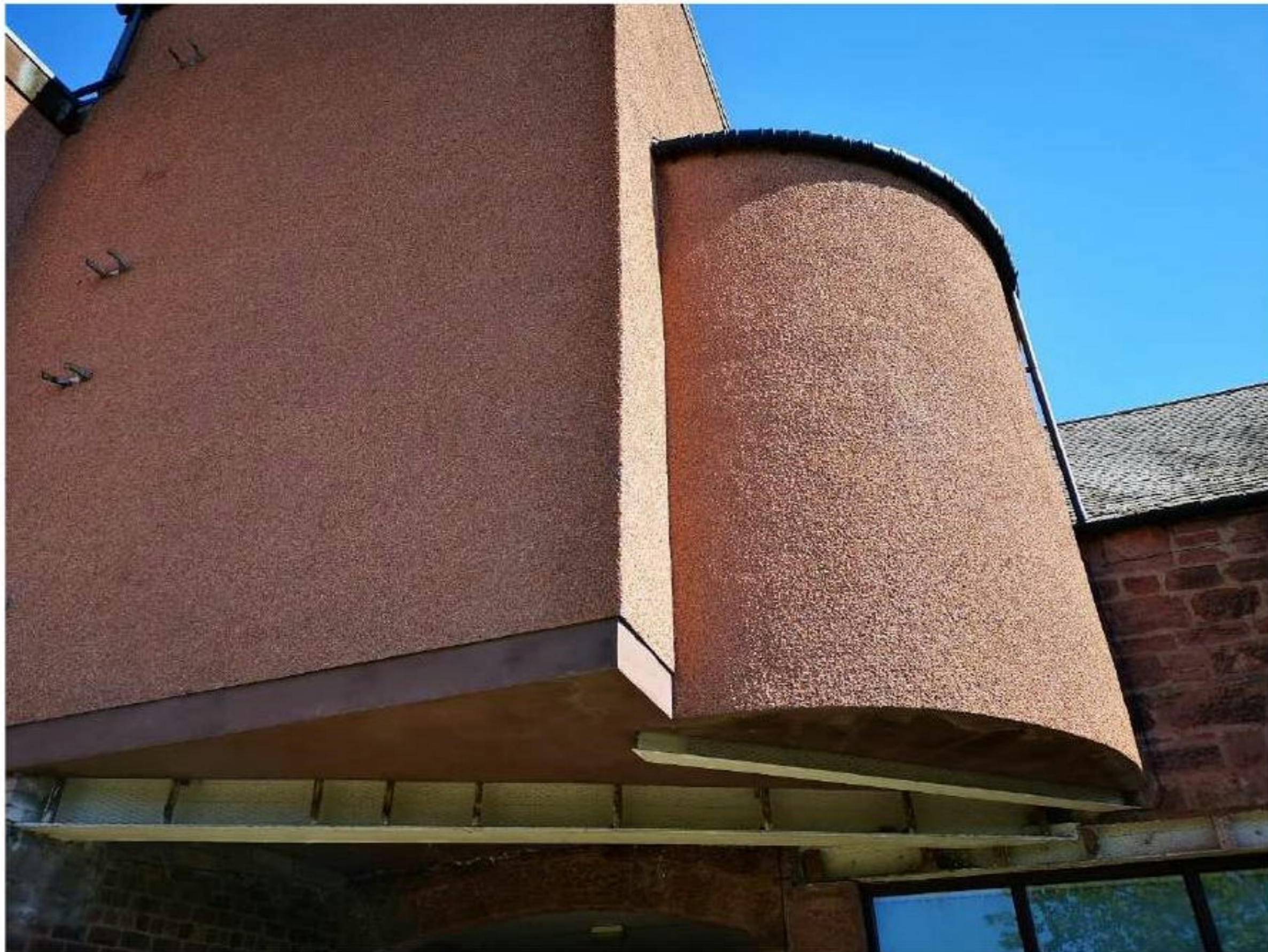
Abbey Theatre building cantilever over pend
