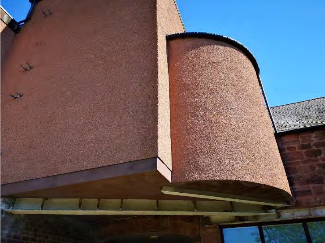
Abbey Theatre building cantilever over pend
