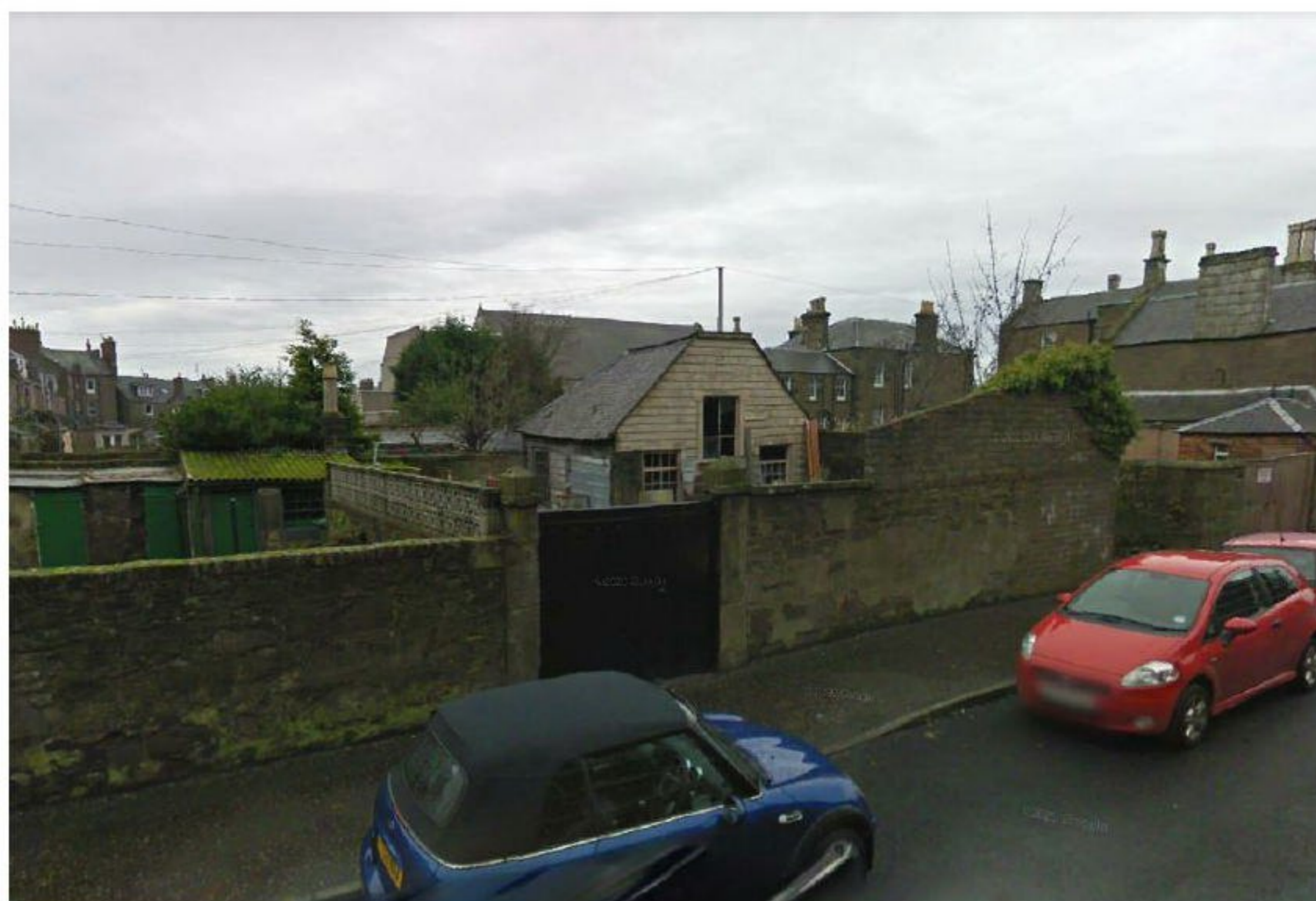
2009 Photo showing existing historic building on site prior to demolition
