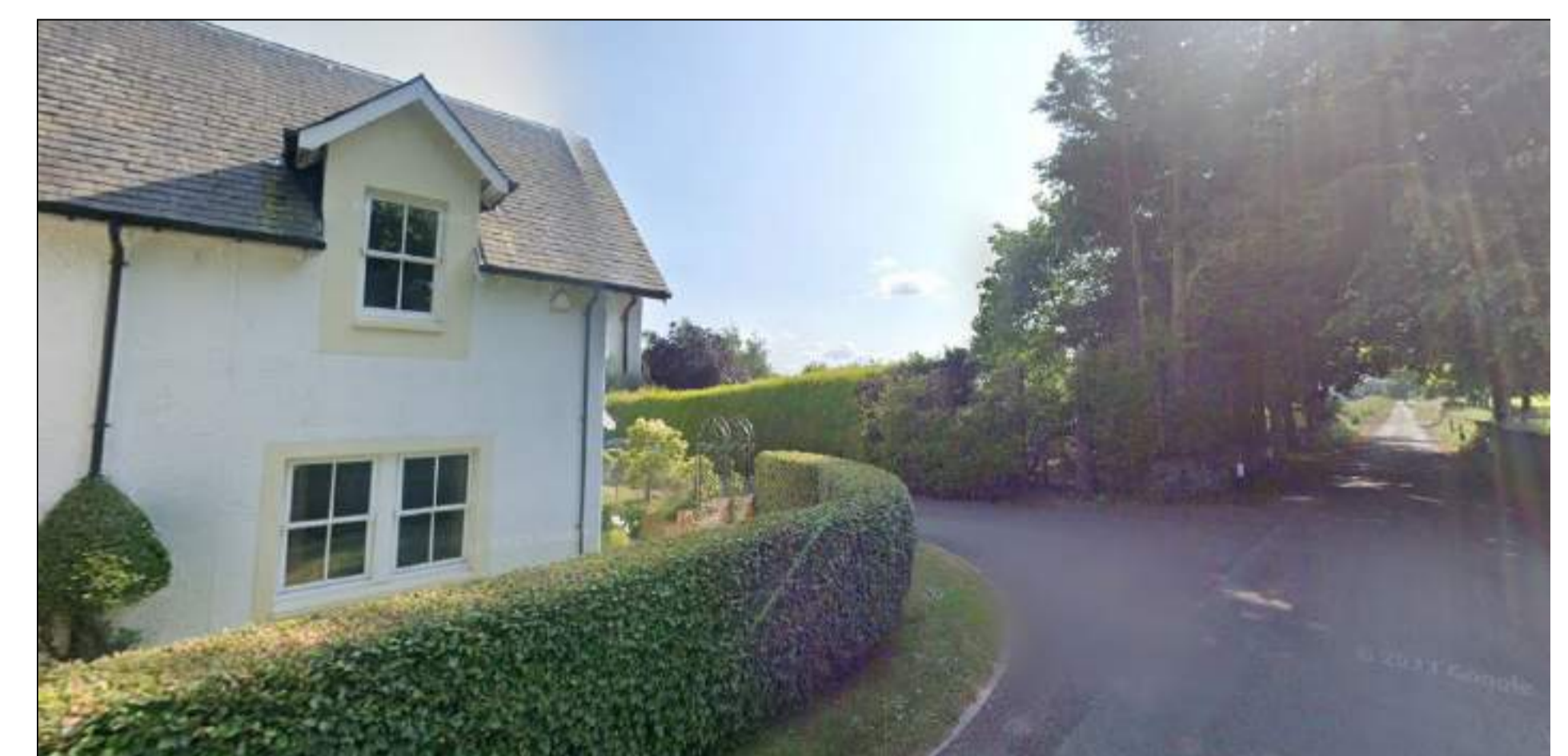
6 - view from East approach
