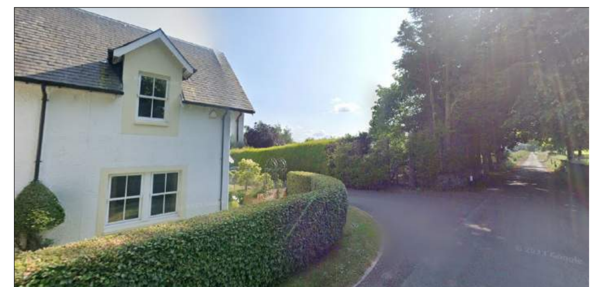
6 - view from East approach
