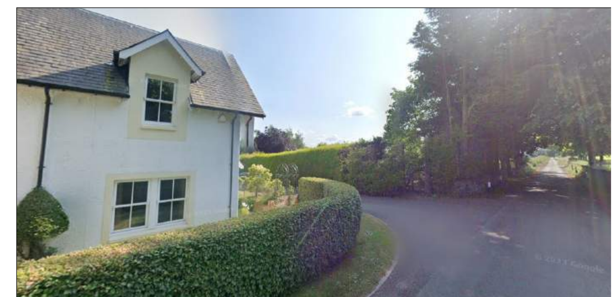
6 - view from East approach
