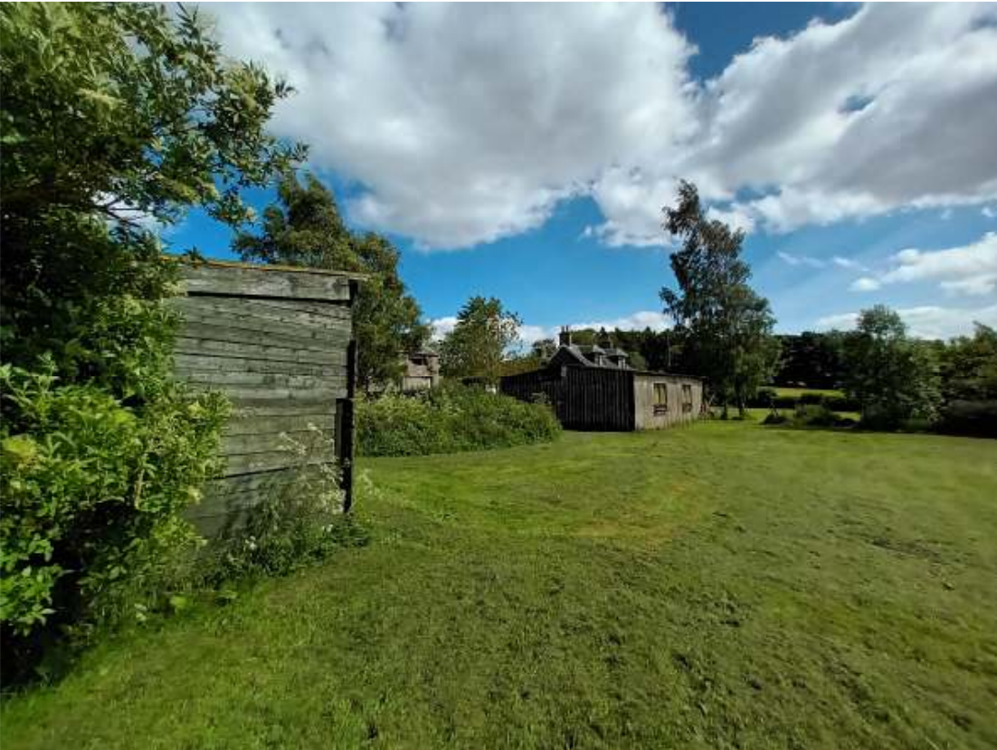
10 View looking South across site
