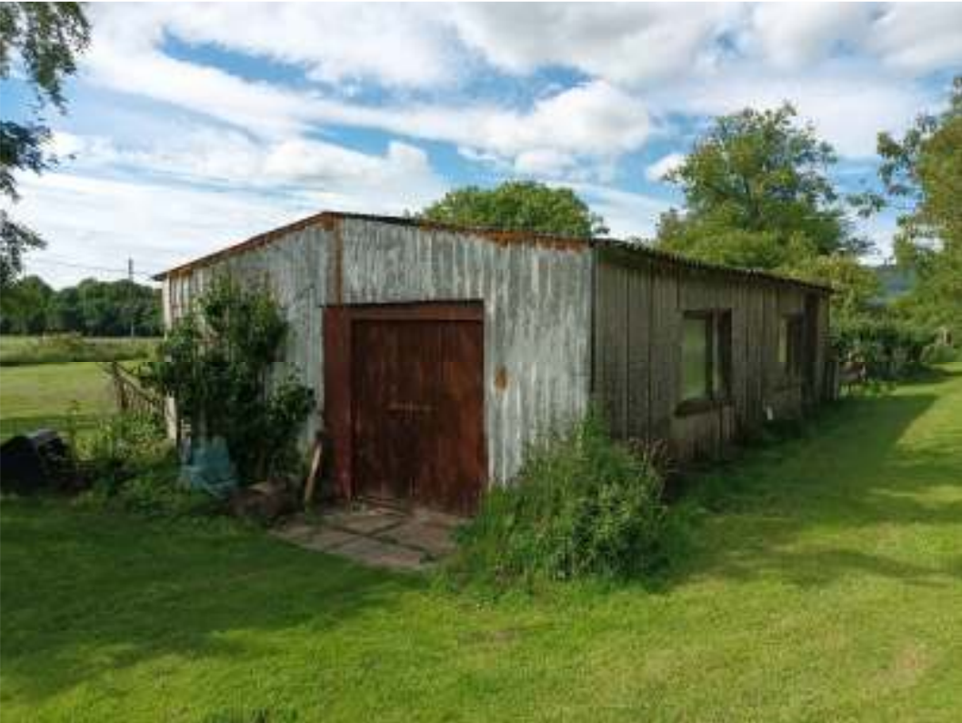
6 Existing Workshop/Storage building
