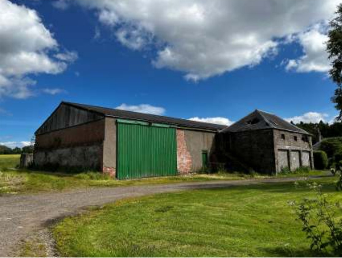
1 View of existing farm buildings to the East of the site
