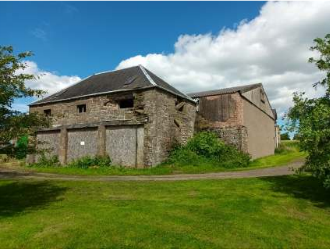
2 View of existing farm buildings to the East of the site
