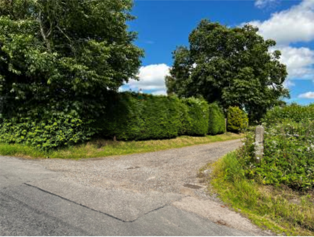
5 Existing access road junction
