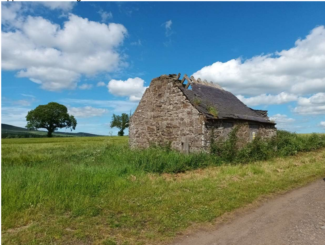
Appendix 3: Ruinous cottage to the North East of the Site.
