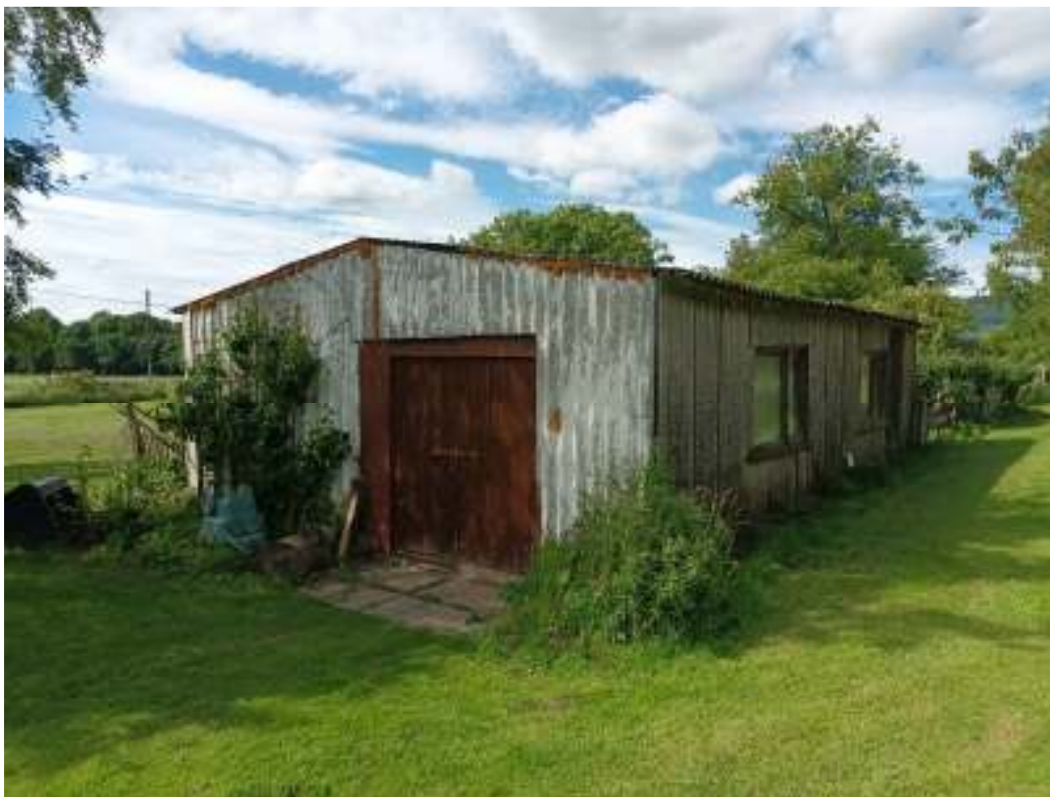
6 Existing Workshop/Storage building
