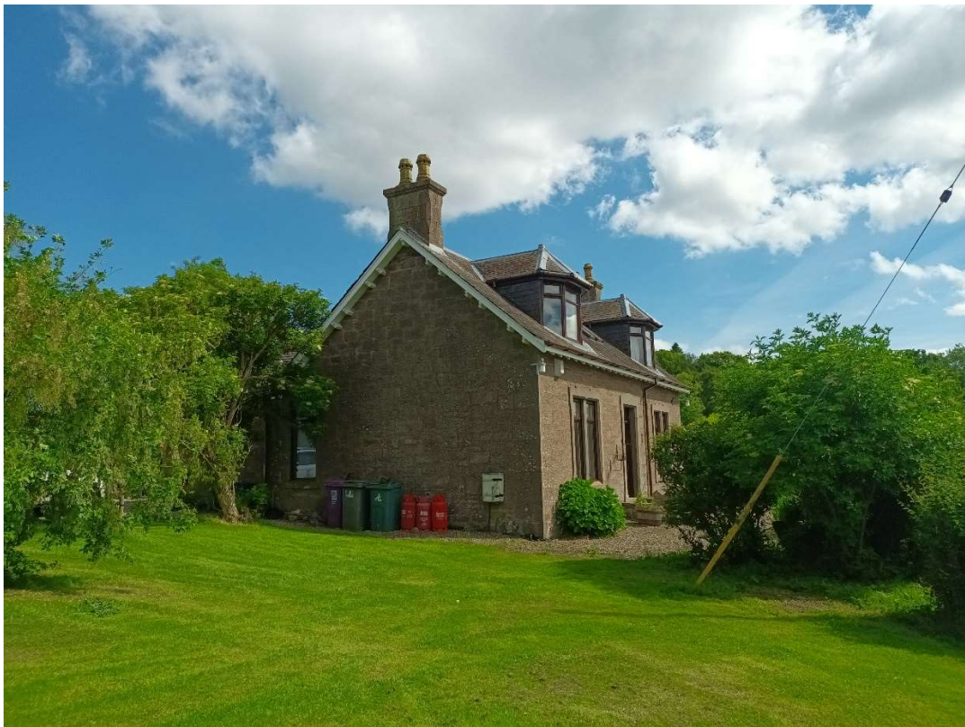
Appendix 5: Gallowhill Cottage
