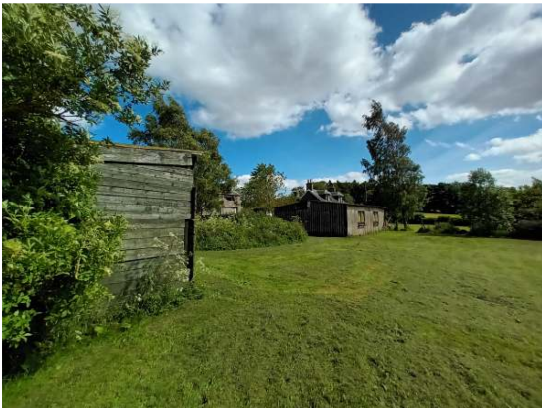
10 View looking South across site
