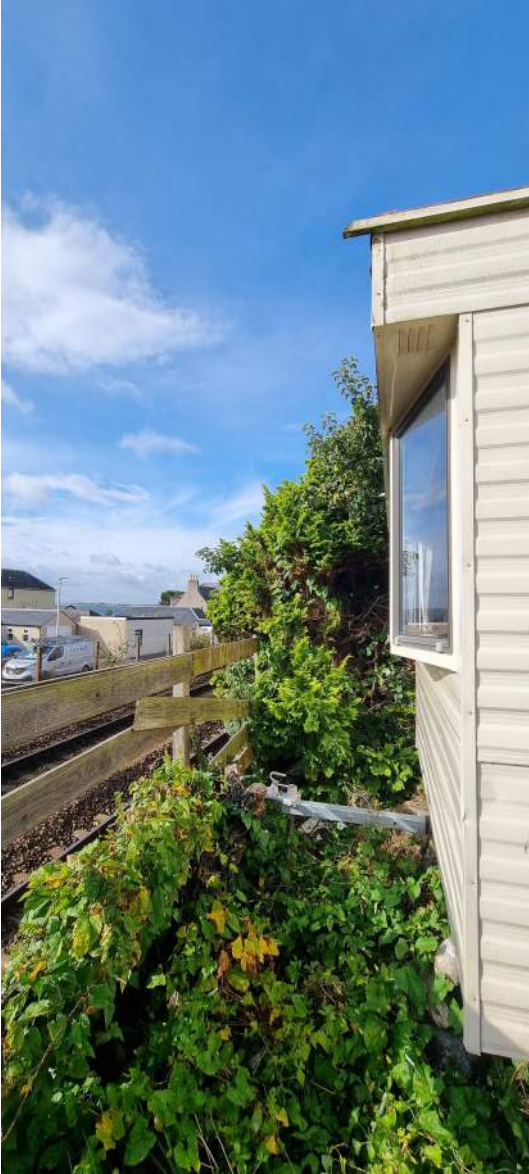
Proximity of caravan to boundary with railway line
