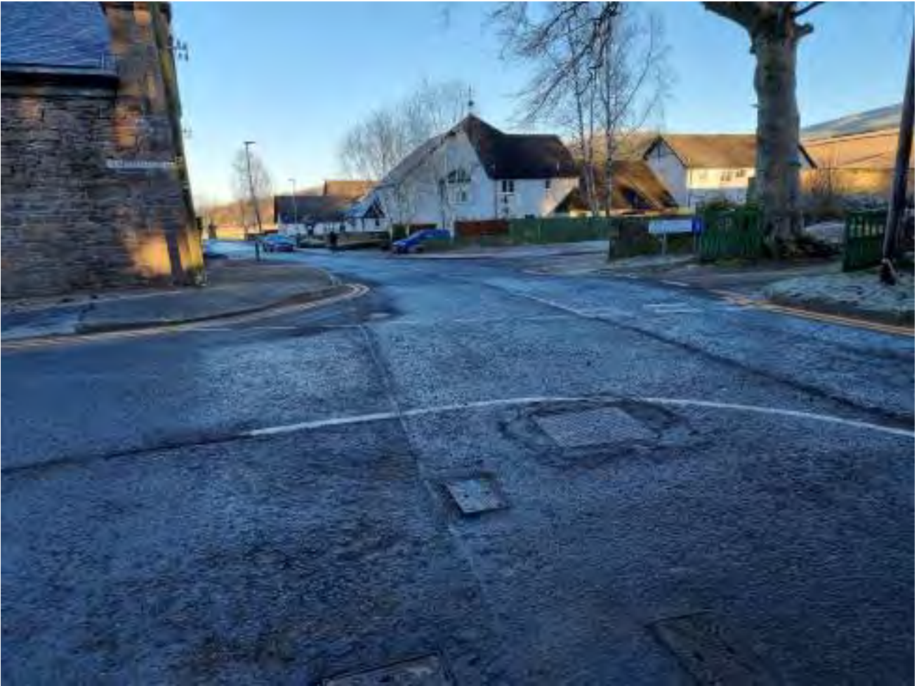
Photograph 6 – looking north east along Knox Close from South Street. The entrance to the culvert shown in Photograph 5 is located in the vicinity of the telegraph pole in the top right of this picture.
