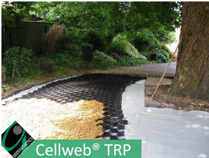
Photo – Cellweb being installed in a tree root protection area.
