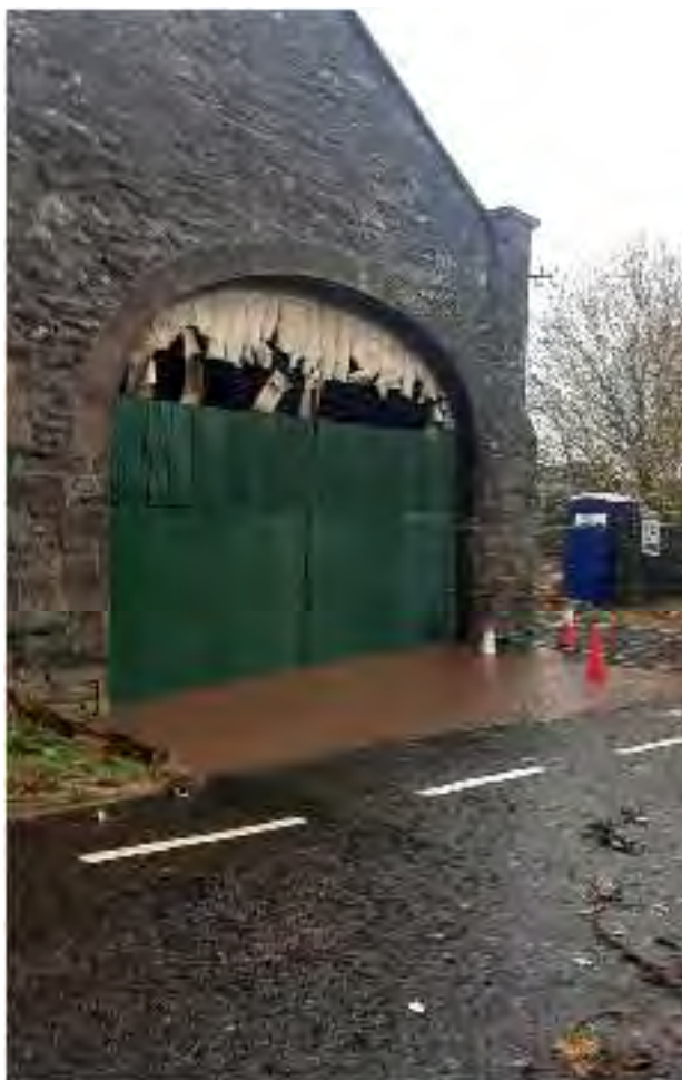
Photo: former train station now residential property corner of south St/ commercial St/ Knox close showing tide line from initial flood.
