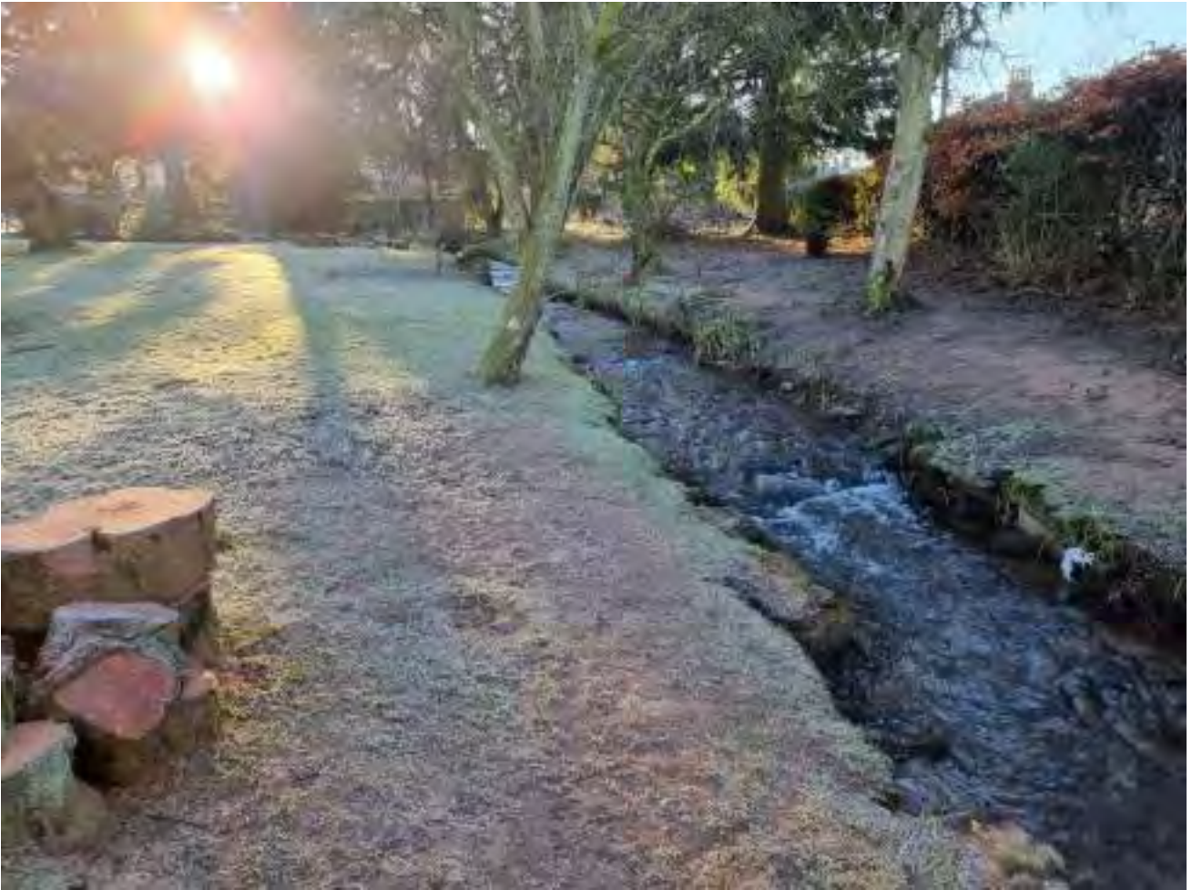
Photograph 4 – looking upstream from the upstream end of the culvert which runs beneath Knox Close. Sediment can be seen on the banks of the watercourse, assumed to have been deposited during a previous high flow event.
